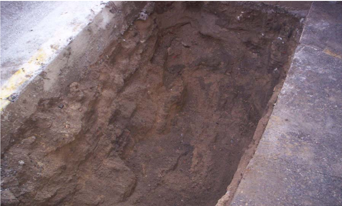
Photo 8: Taken south to north. Shows completion of test pit #2 with no utilities present.
