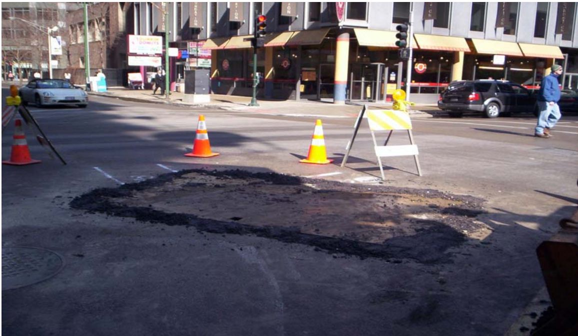
Photo 6: Taken east to west. Shows placement of steel plate over test pit #1 after its completion.
