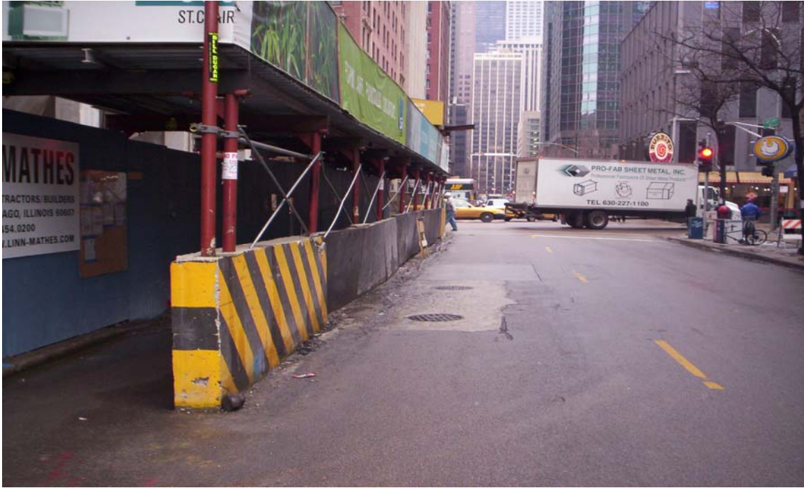
Photo 1: Taken south to north. Shows locations of planned test pits along St. Clair near alley and looking north towards Ohio prior to beginning work.
