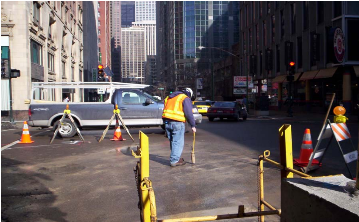
Photo 3: Taken south to north. Shows radiation walkover survey above location of test pit #1 prior to beginning excavation.
