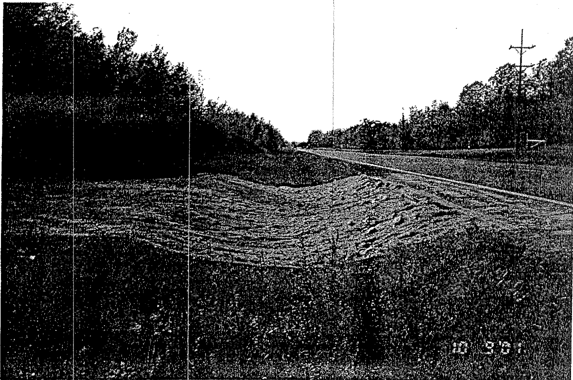
Completed Excavation, Looking West
