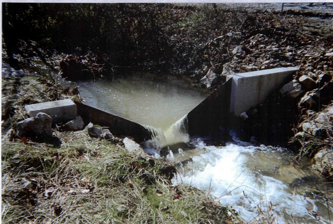
Photograph No. 12 Orientation: Southwest Description: Overflow at V-notch weir in Conard's Branch
