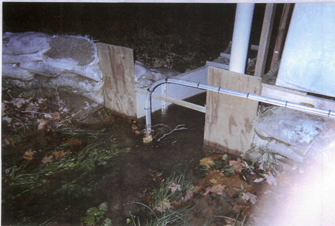
Photograph No. 19 Orientation: Northwest Description: Overflow at V-notch weir at Overflow Spring 0
