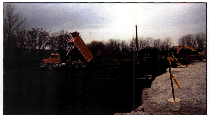
Backfill of Excavation Areas
