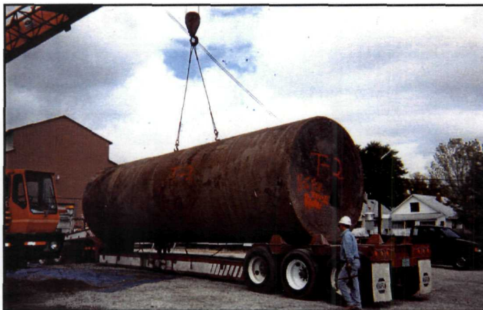
Off-site transport of UST
