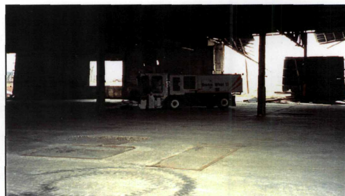
Final Decontamination Using Dry Vacuuming Unit
