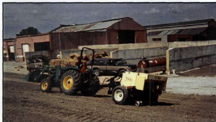
Installation of Native Prairie Vegetation
