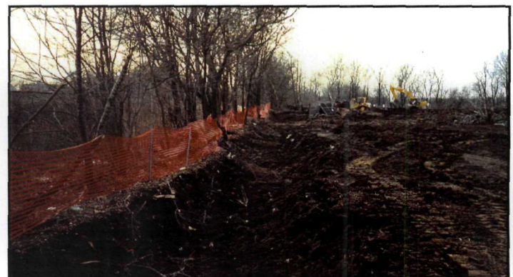
South Property Boundary Excavation
