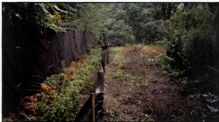
Silt Fence Installation
