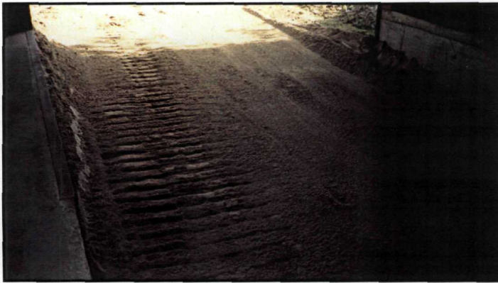
Interior Rail Spur Backfill
