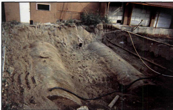
UST Removal Activities
