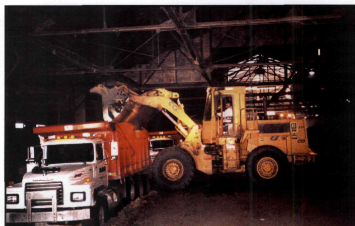
Loading of trucks with residential soil in the East Warehouse at the Avanti Site
