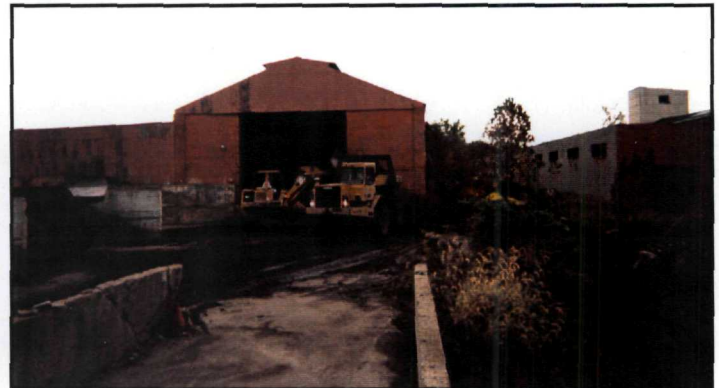
West Warehouse Loadout Operations
