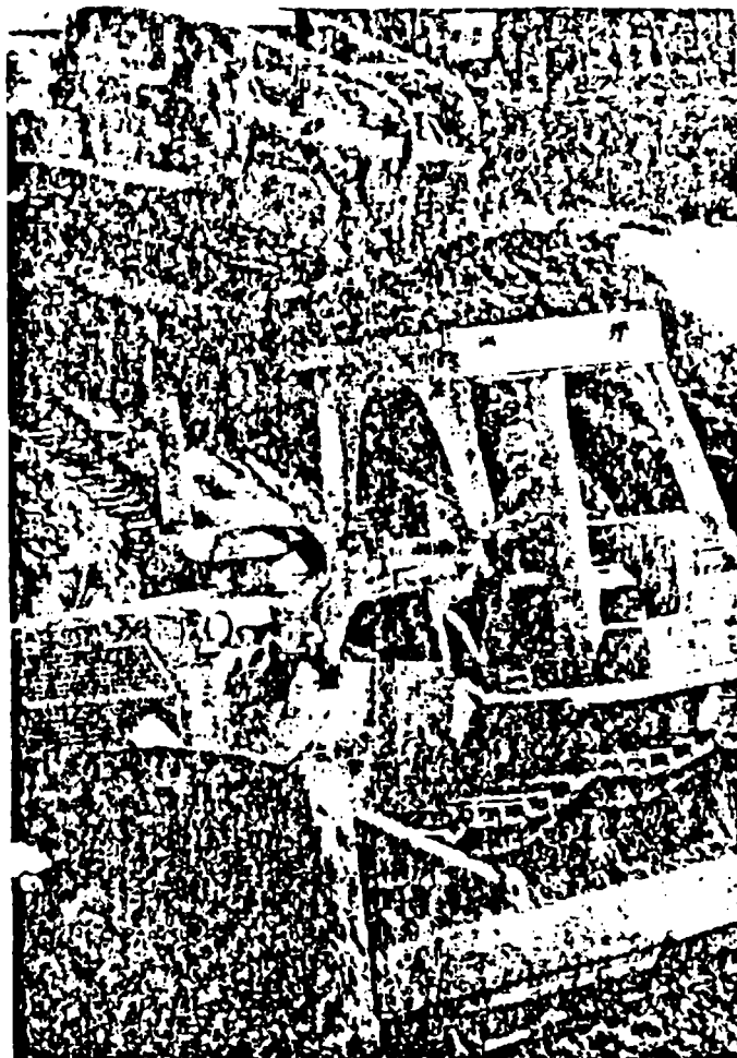
Bulldozers sealed contaminated soil into a 30-foot deep "containment area" lined with clay and plastic.
