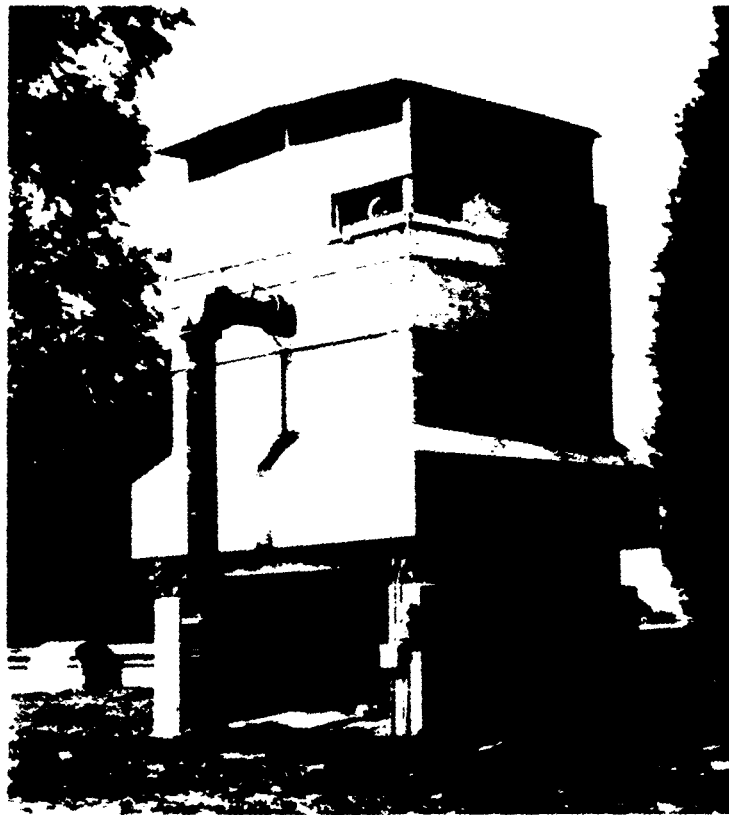
DETOX Air Stripper Wright-Patterson AFB
