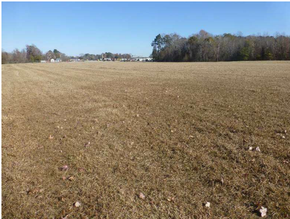
View of the grass-covered part of the OU-1 cap, looking northeast
