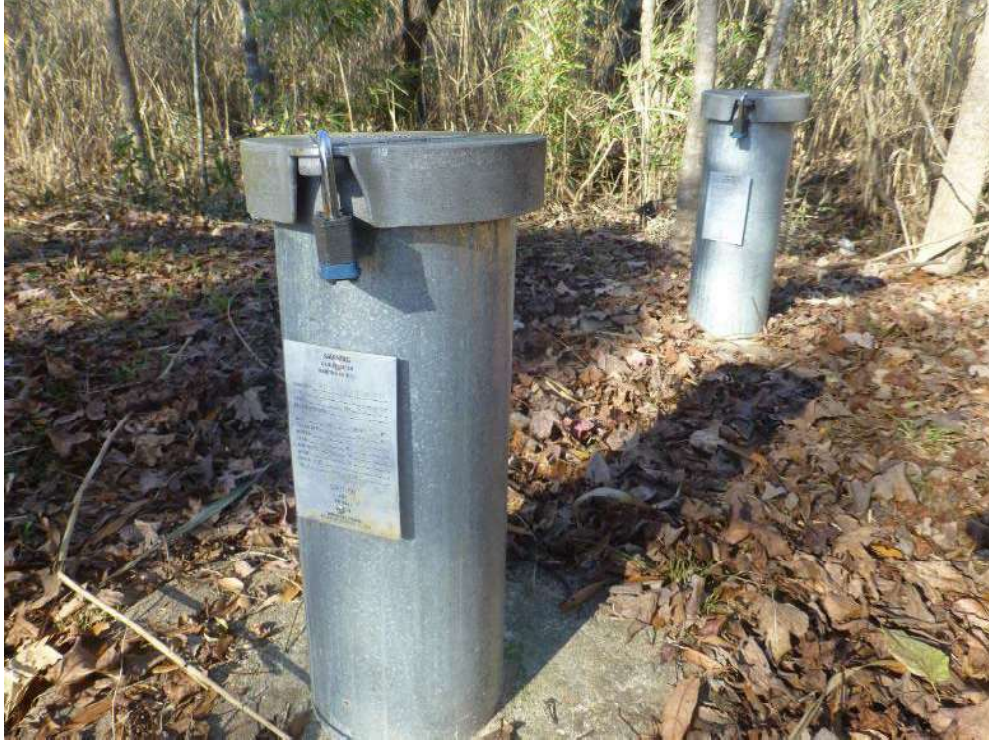
Wells FL-10-1 and FL-10-2, outside the northern edge of the OU-1 landfill cap
