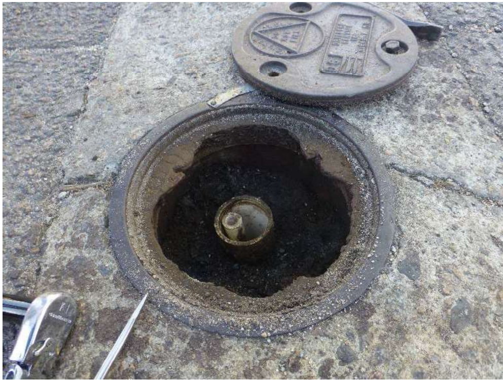
Flush-mounted groundwater monitoring well at OU-3
