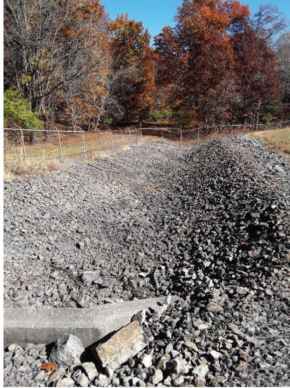
Riprap channel to the east of the back gate, looking east.
