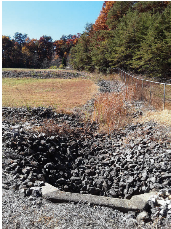
Riprap channel to the west of the back gate, looking west.
