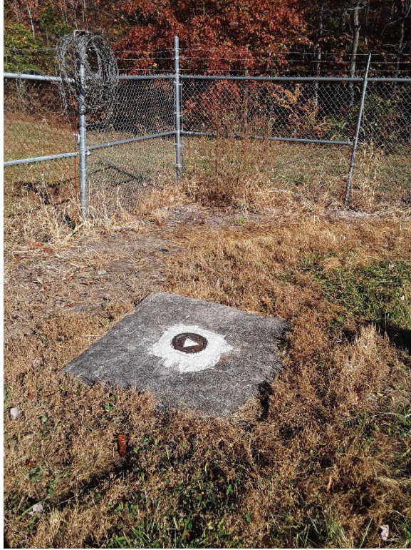
ATL-8 was damaged during mowing in 2020 and was revamped into a flush mount configuration.
