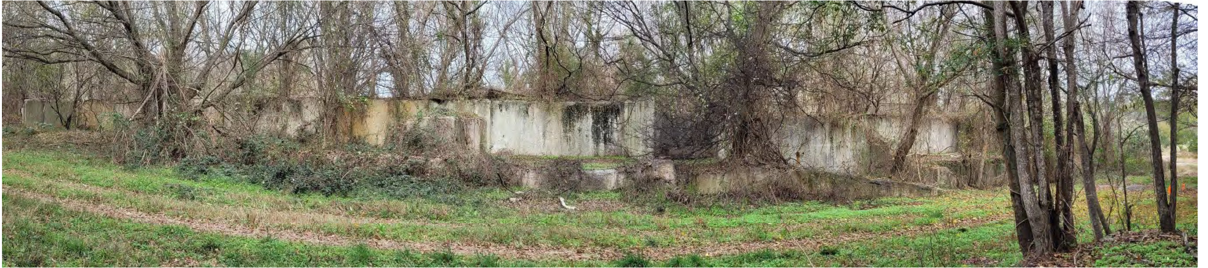
Site Photograph N2 – Foundations for Former Process Buildings
