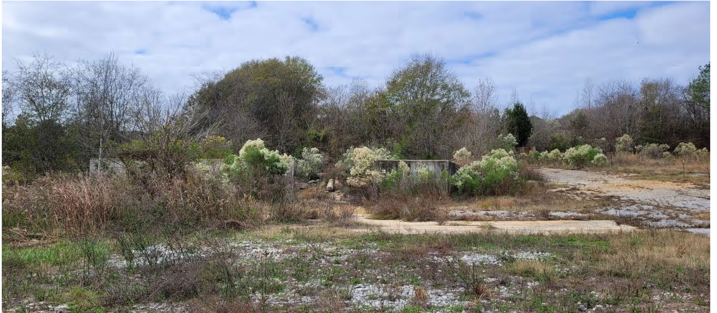
Site Photograph N3 - Foundations for Former Process Buildings from East Looking West
