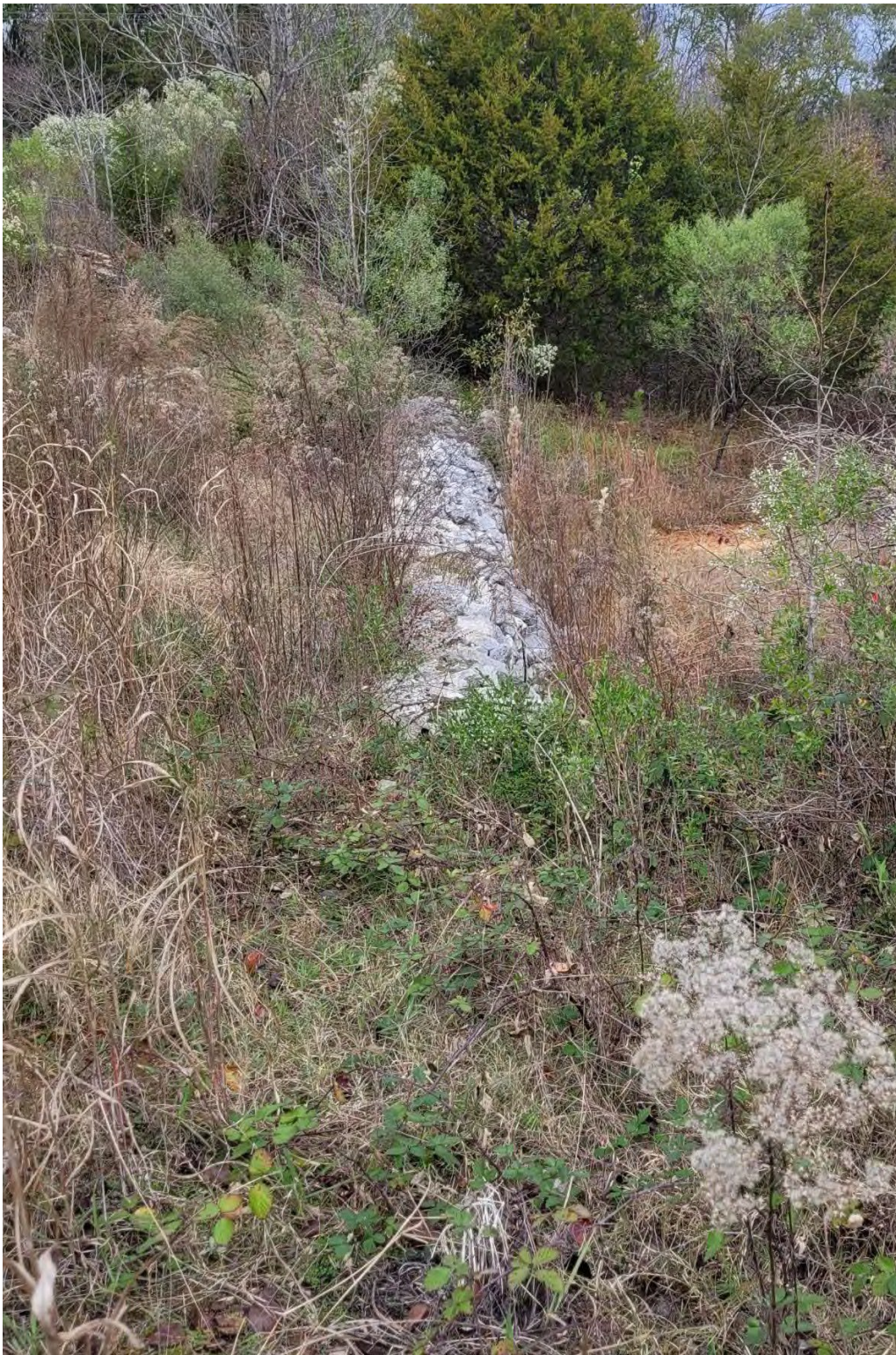
Site Photograph N5 - Rock Check Dam (East of Infiltration Area 2)
