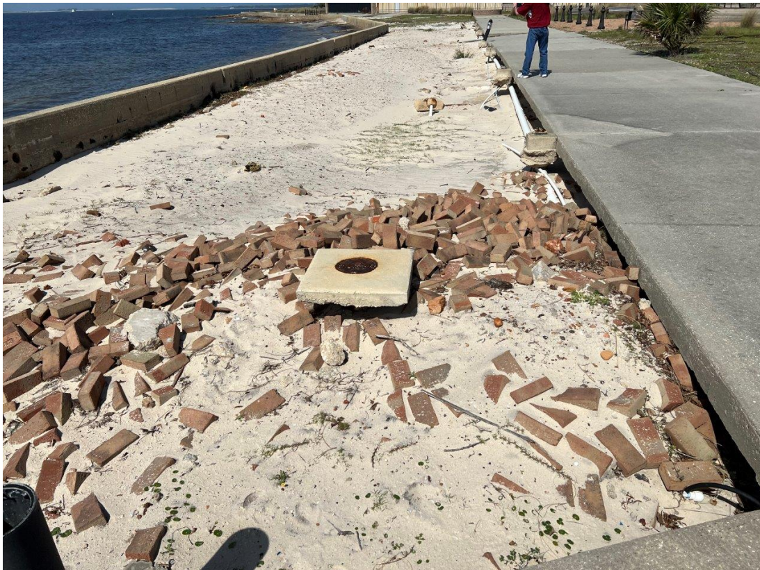
OU 11 Site 38 Former Building 71 shoreline looking north at well 38GS13
