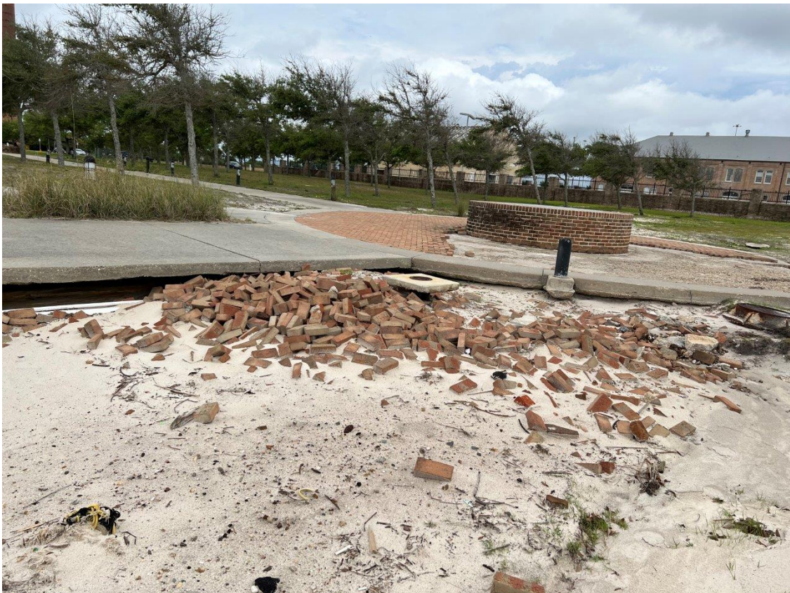
OU 11 Site 38 Former Building 71 shoreline east of gazebo
