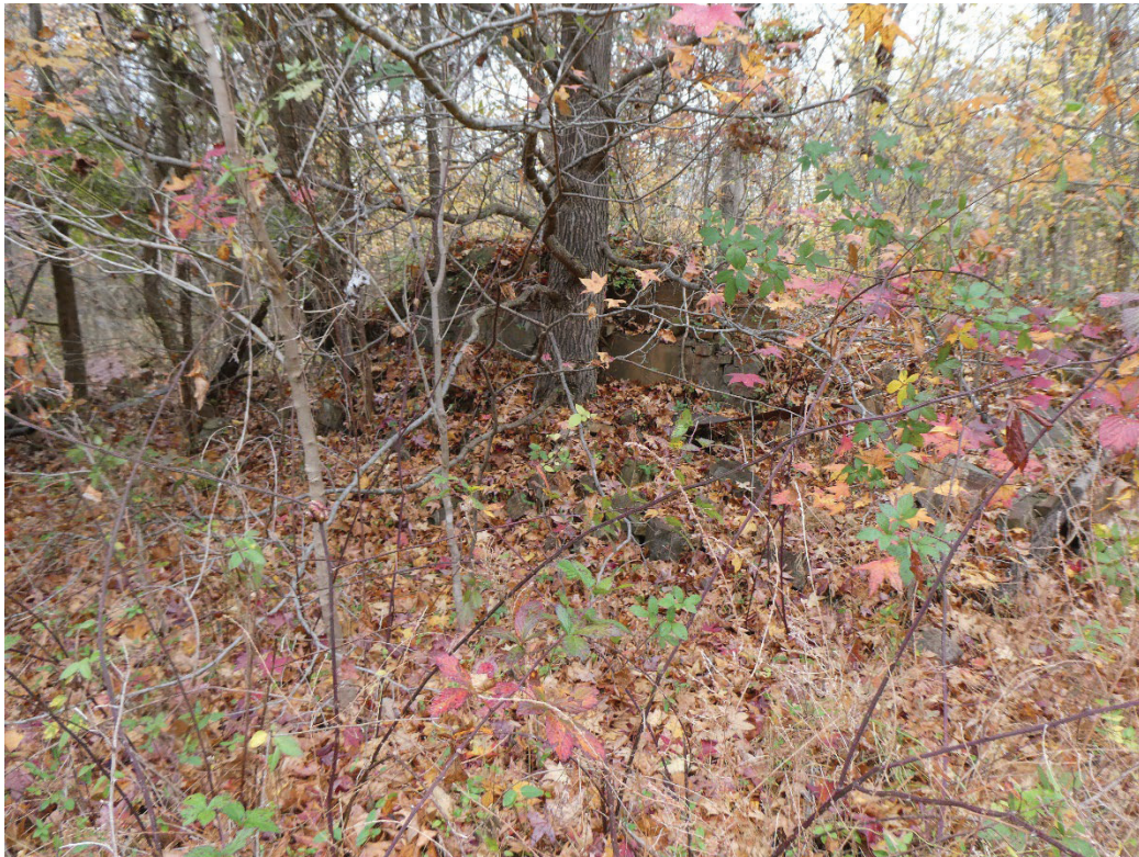
Deteriorating brick formations from former operations
