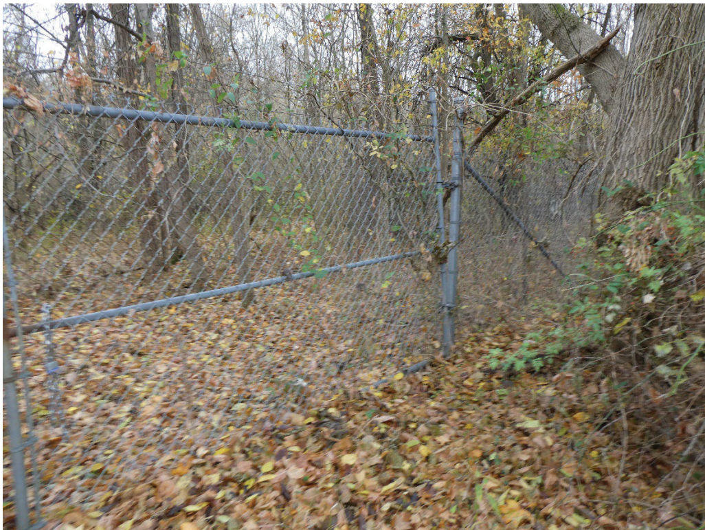
Secured gate along road
