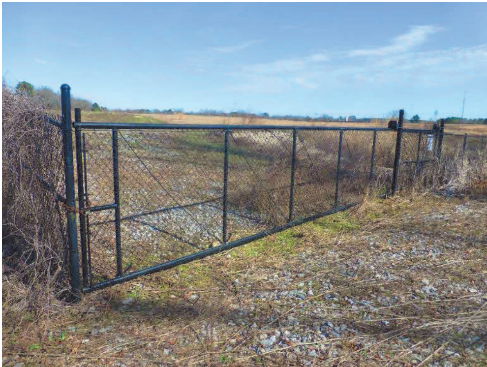
Locked gate at entrance to capped areas
