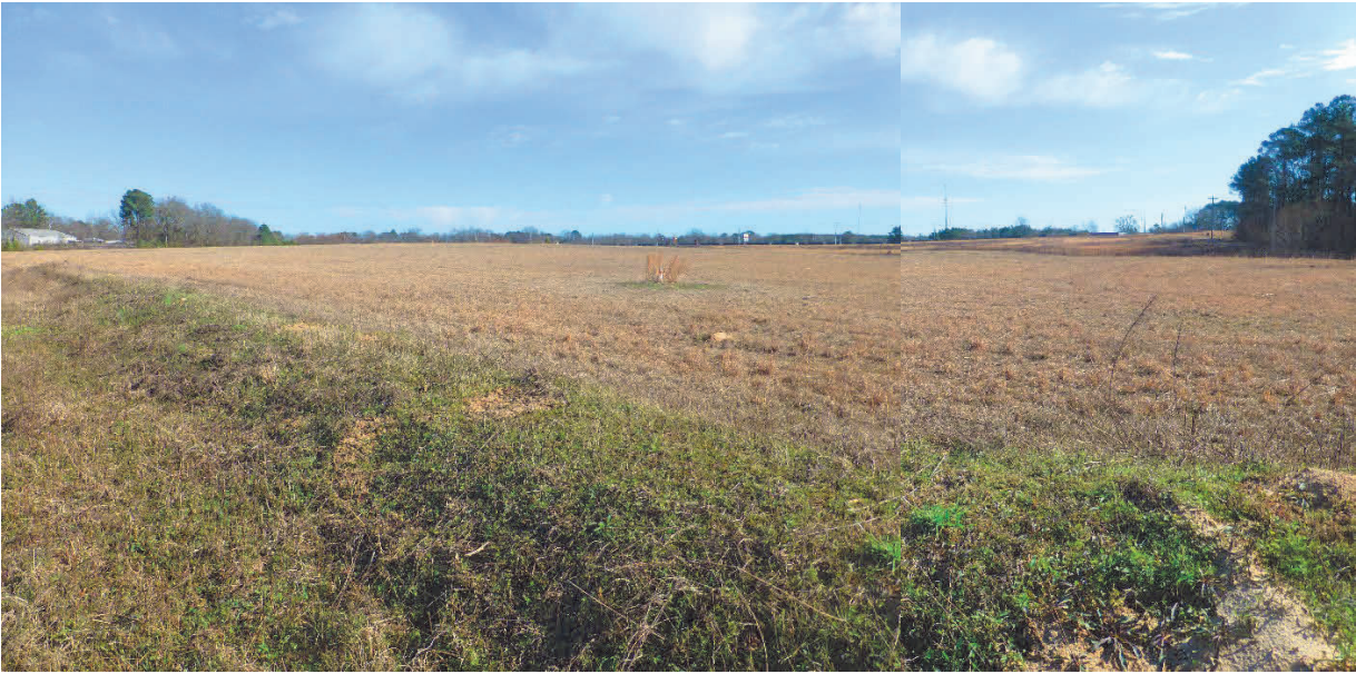
Capped containment cell, looking northeast
