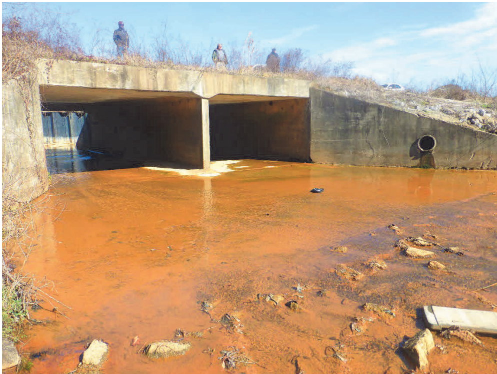
Baremore Street culvert
