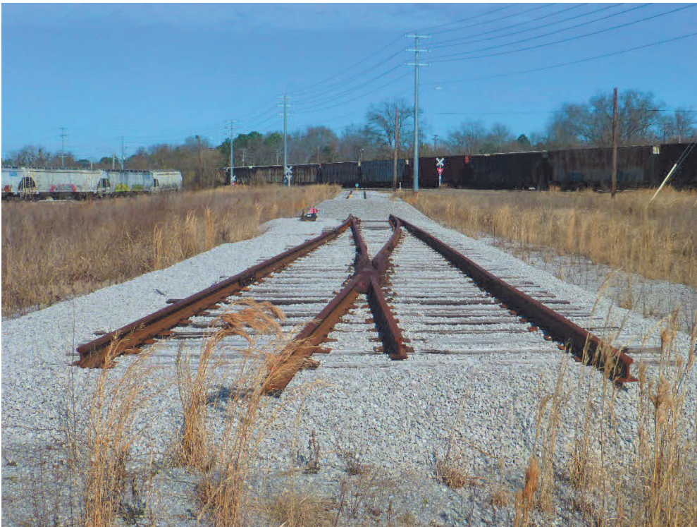
Rail spur on northern part of the Site
