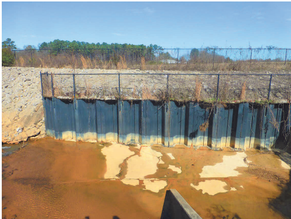
Sheet piling wall at Baremore Street culvert
