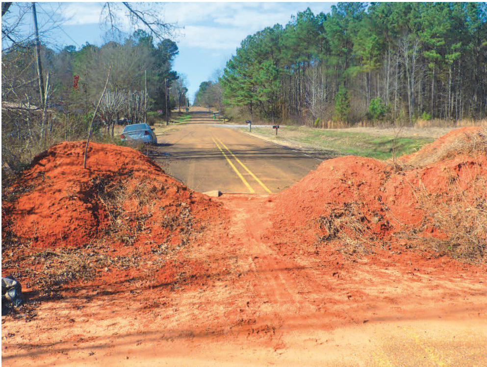
Baremore Street, near culvert, looking west
