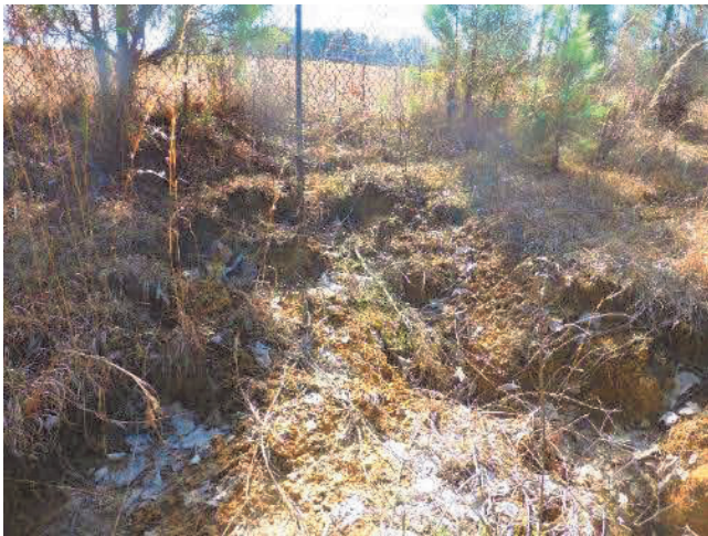
Eroded areas between the northern edge of the capped containment cell and the creek (near Warren Chapel)
