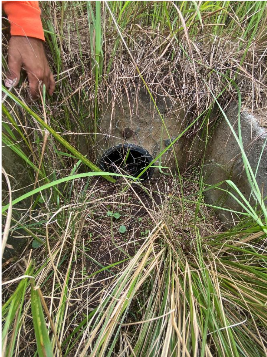
Landfill letdown pipe located at toe of landfill berm
