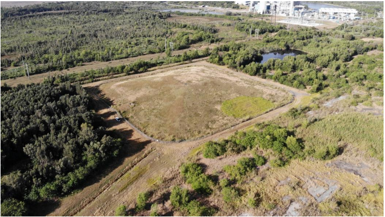
Drone photo looking west across landfill toward stormwater pond
