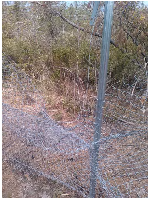
Close-up of fence damage south of Old Sawmill Road at Site 74.
