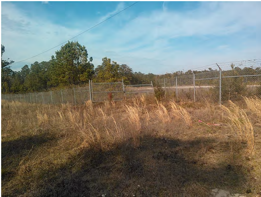
Damage to fence along Defense Reutilization and Marketing Office (DRMO) at Site 6, facing east.
