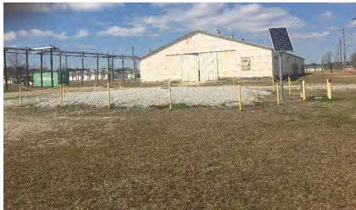
Solar panel at Site 93, facing north.
