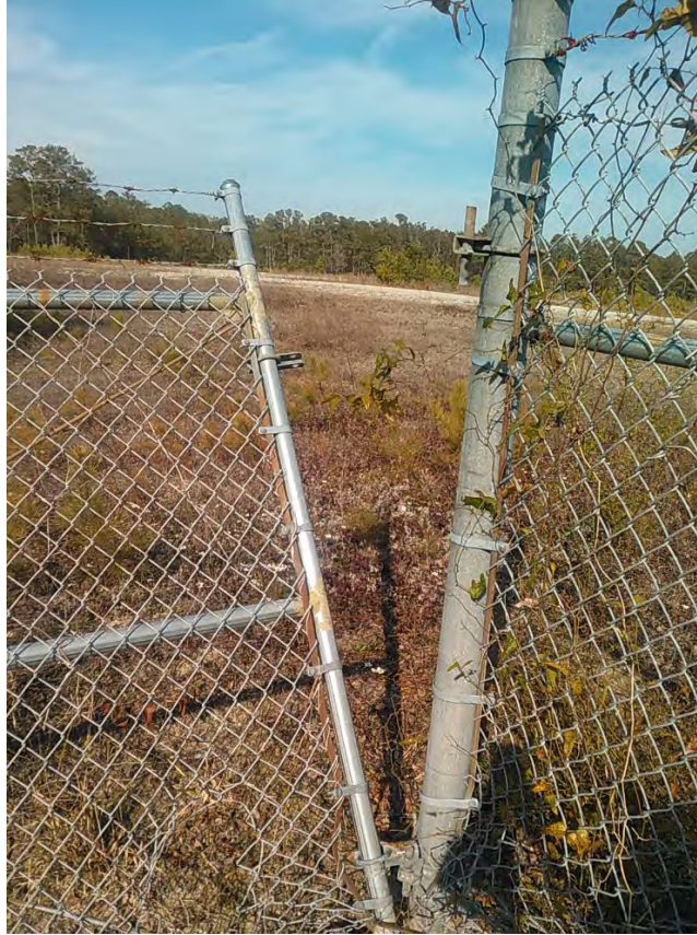
Closeup of fence damage at Site 6, facing E.
