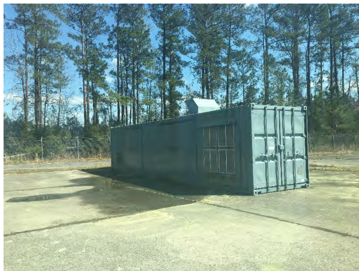
Sparge system at Site 89, facing southeast.
