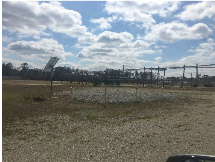
SBGR at Site 93, facing southwest.
