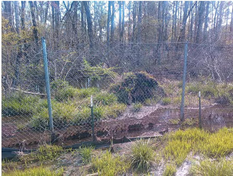
Damaged fence near first aerator east of White Street at Site 89, facing south.
