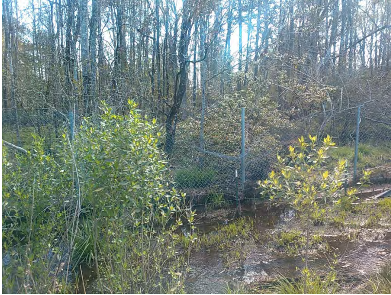
Damaged fence along Edward Circle at Site 89, facing south.
