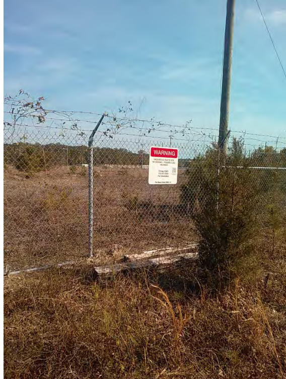
Warning sign near damaged fence along DRMO at Site 6, facing east.
