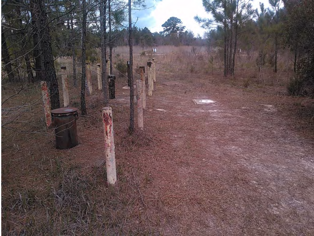
IR03-MW02 cluster at Site 3, facing north.
