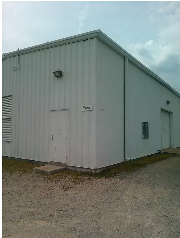
Building 976A North treatment plant at Site 78, facing northwest.
