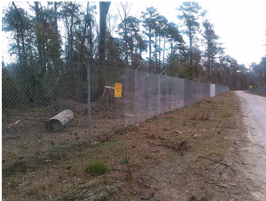
Fence at Site 74, recently repaired from hurricane damage, facing southeast.
