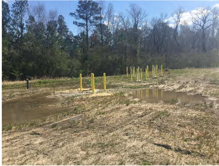
New wells at Site 89 in former DRMO area, facing south.
