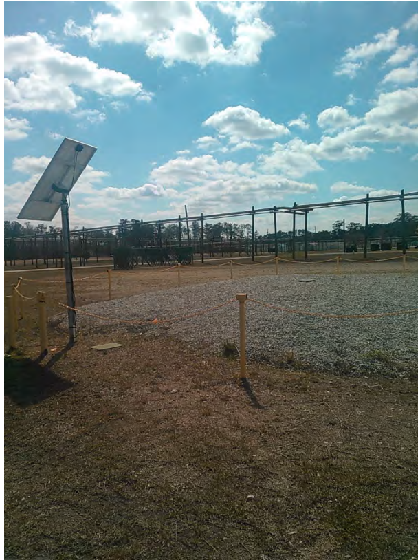
SBGR at Site 93, facing southwest.
