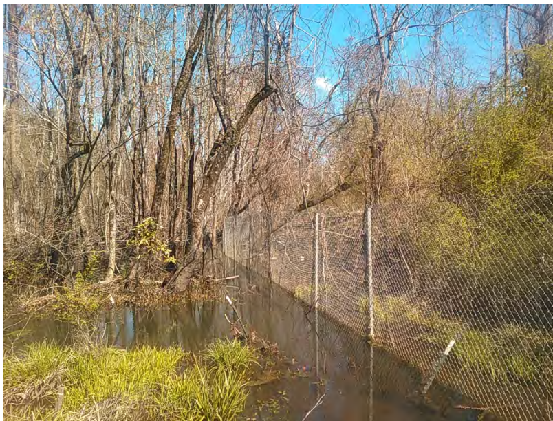
Ponding edge of clearing and PRB-B and tree down at Site 89, facing east.
