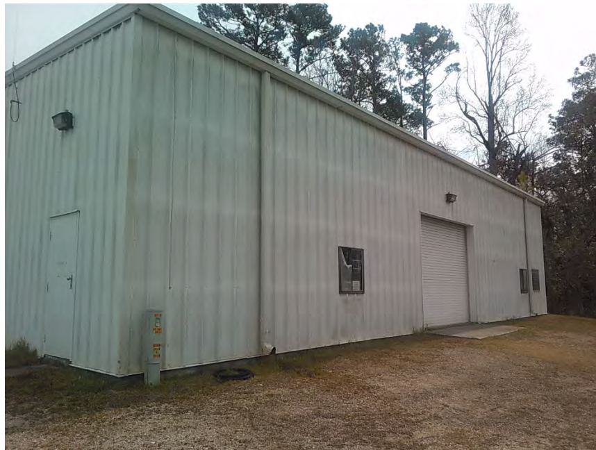
South treatment plant at Site 78, facing south.
