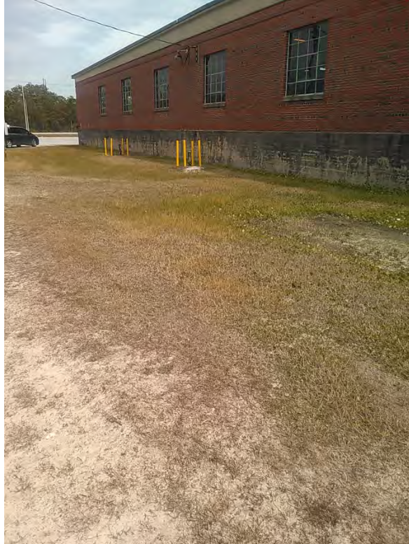
Building 903 at Site 78, facing east.
