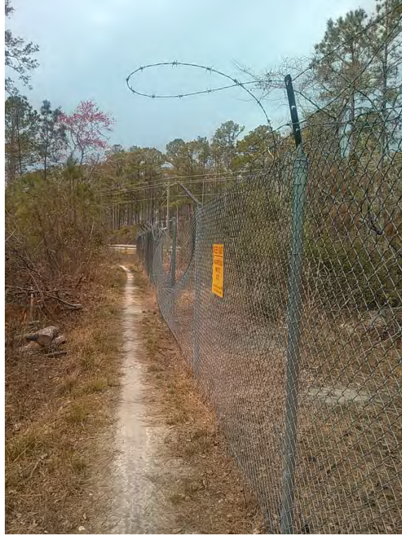
Fence south of Old Sawmill Road at Site 74, damaged fence visible, facing northwest.
