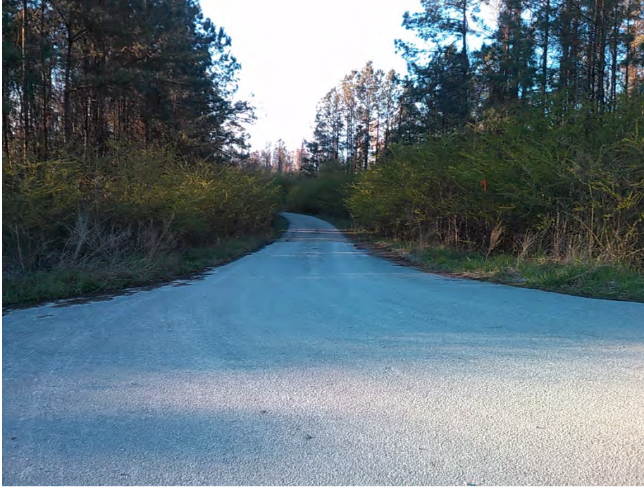
Access road at Site 36, facing south.
