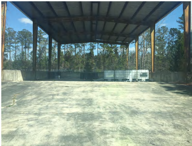
Storage area within former DRMO area at Site 89, facing east.
