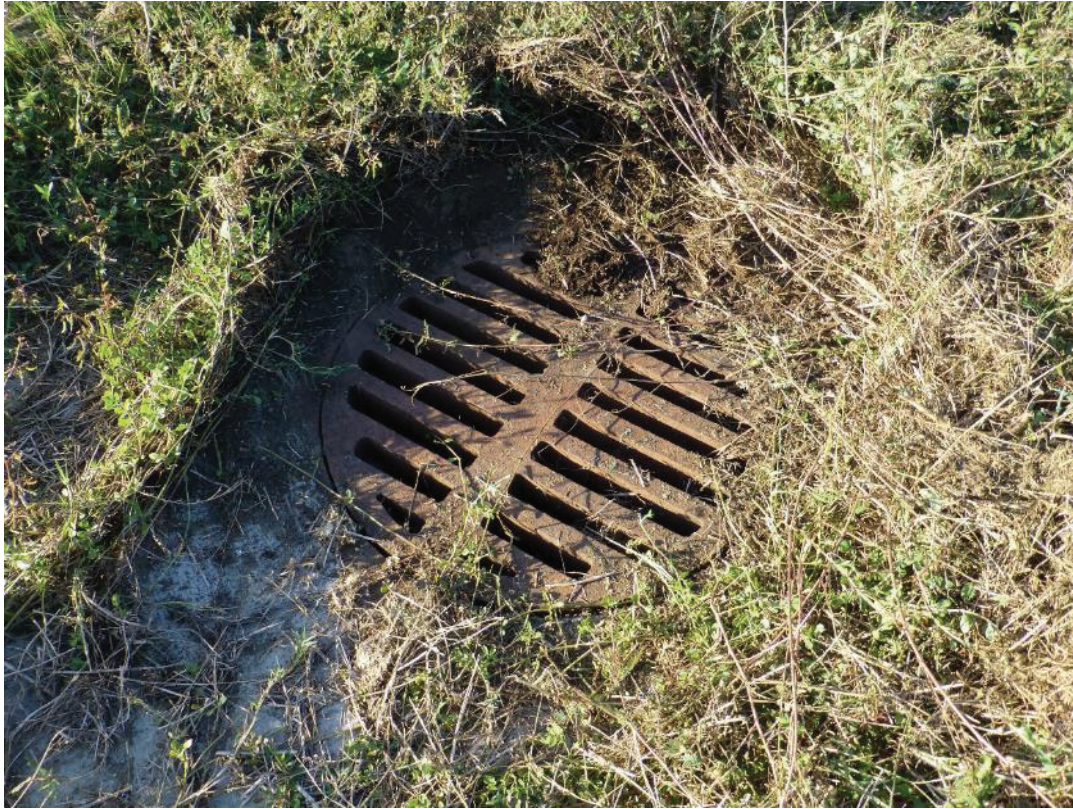
Stormwater drain on the southern part of the Site
