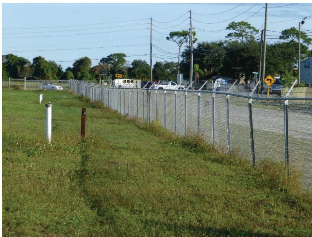
Fence and monitoring wells along Anclote Road on the southern part of the Site
