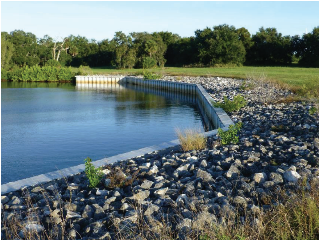
Seawall and riprap along Meyers Cove (southwest side of the Site)
