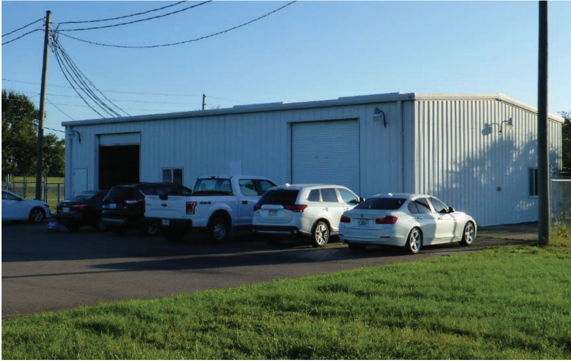
On-site maintenance building (used for current site maintenance)
