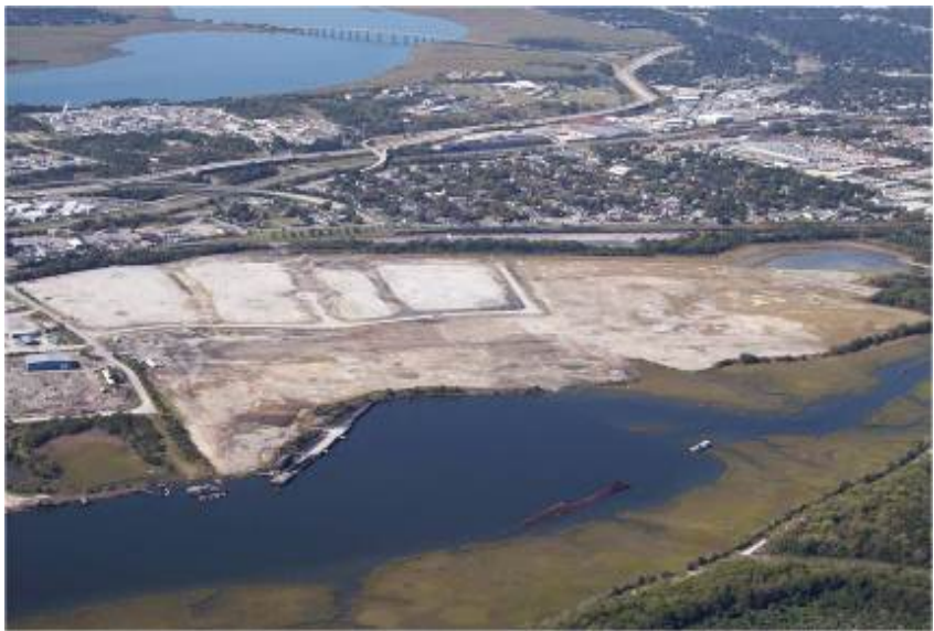
Figure 3: Macalloy Corporation Superfund site following cleanup activities
