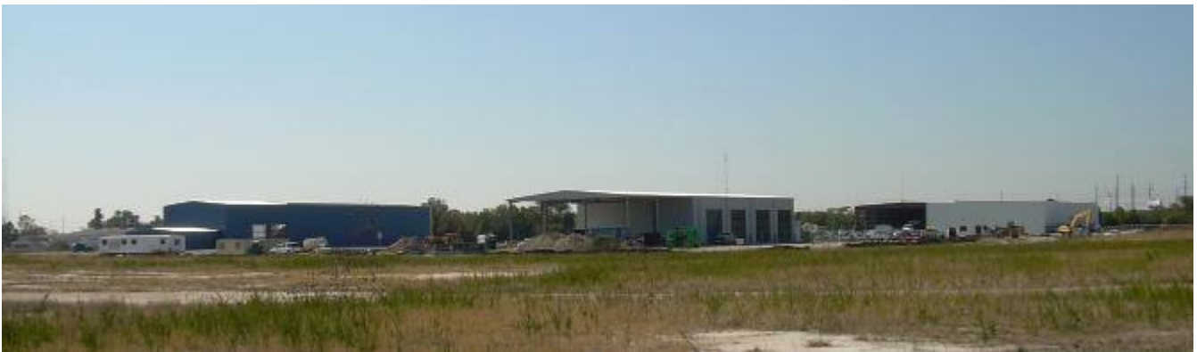
Figure 4: The 30-acre industrial park located on the southern portion of the site
