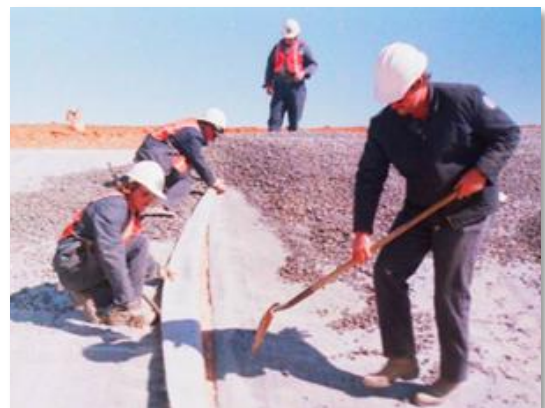
Figure 3. Workers install recycled tire chips as part of the landfill cover.
