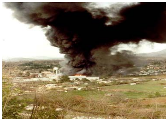
Figure 4: A fire in 1982 destroyed Benfield Industries' chemical plant at the site. (Source: EPA)
