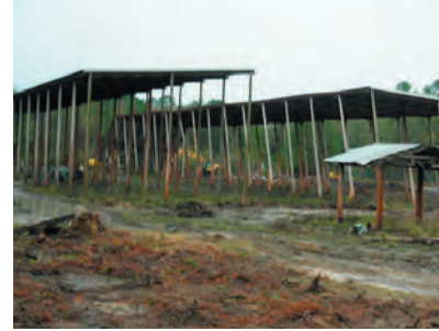
Pole barn #1 prior to demolition. 1/22/2007
