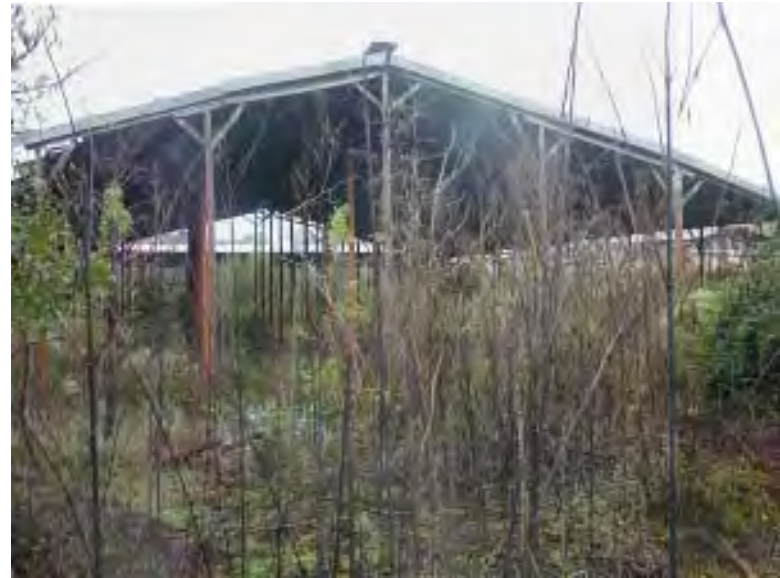
View of remnant pole barns
