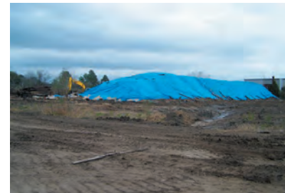
Drip Track Stockpile in the Northeastern Area of the Site. 1/30/2007
