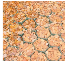
INTERLOCKING MESH WITH GRAVEL (ABOVE) AND GRASS (LEFT) SERVE AS A POROUS PAVER ABLE TO WITHSTAND VEHICULAR LOADS
