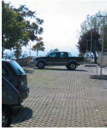
POROUS BLOCK PAVING EXAMPLE
