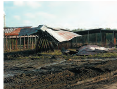
View of pole barn #4 being pushed over with the Kobelco excavator. 2/7/2007
