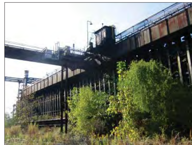
Coke Battery Building
