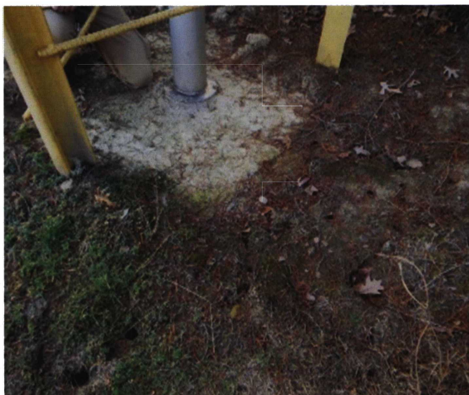
Padding on well ALT-1 buried under a soil layer
