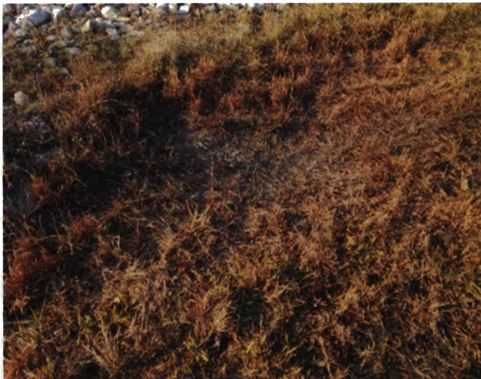
Settling of the cap observed in the middle portion of the capped area
