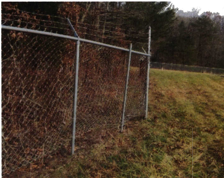
Slightly broken security fence in the north and growing tree limbs on the fence
