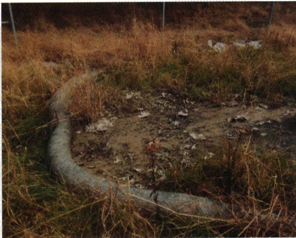
Berms and socks installed to control runoff from the draining ditch near fence line in the southeast portion of the Site
