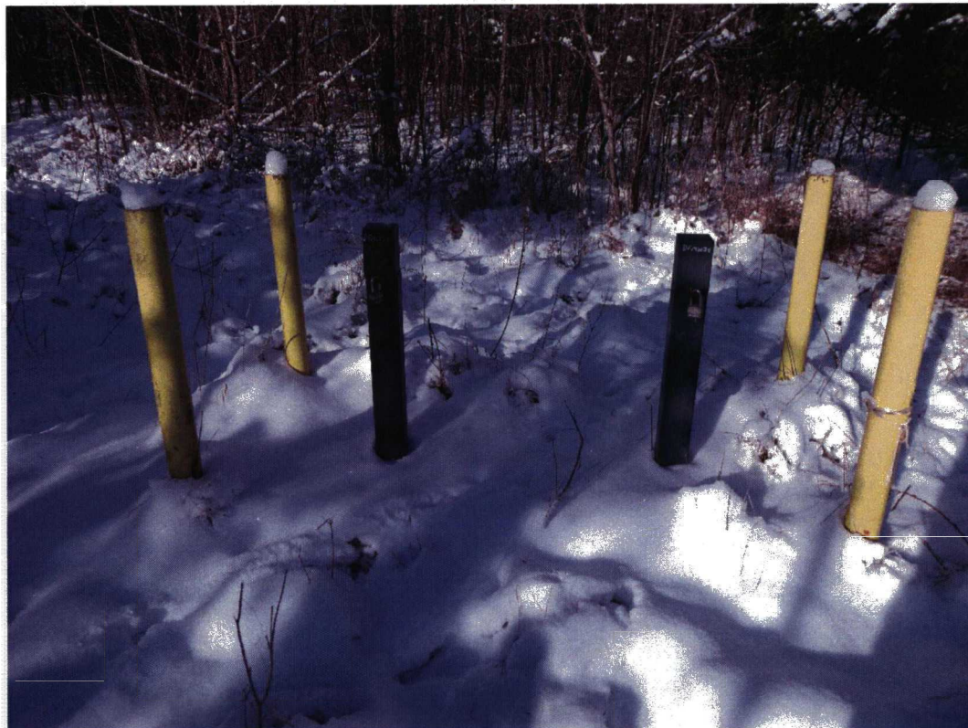
New wells DFMW-3S and DFMW-3D
