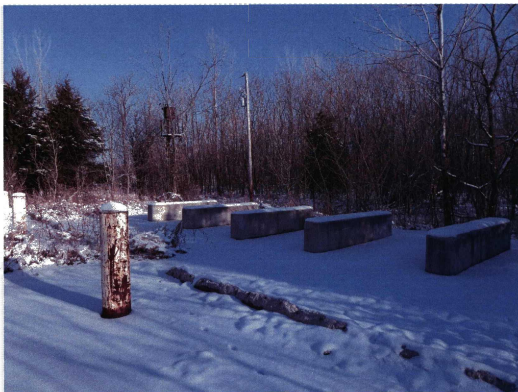
Location of former building and tank
