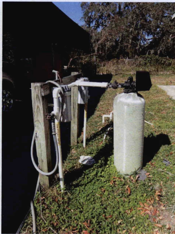
Inactive carbon filtration system on private well (now used for non-potable purposes)
