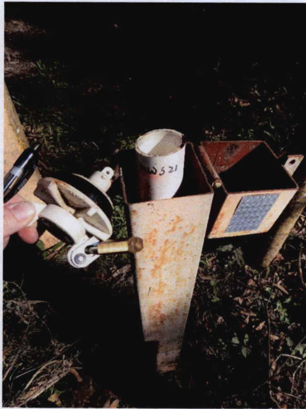
Unlocked monitoring well MWS-21
