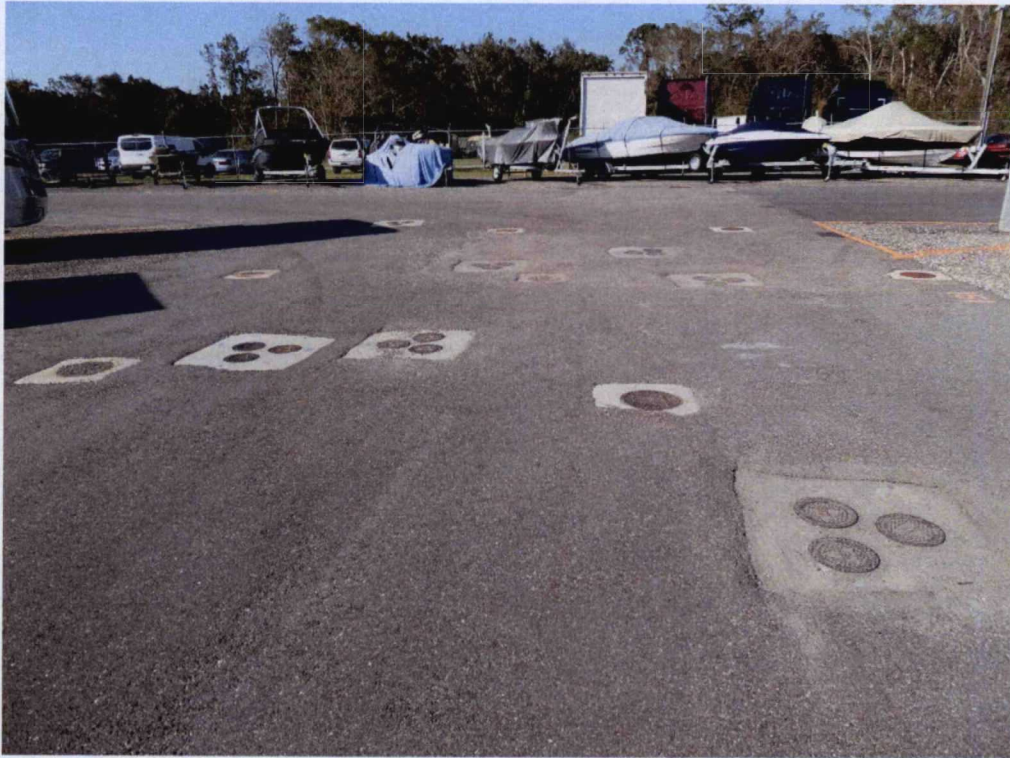
Looking southwest from relict sinkhole area with flush-mounted monitoring wells visible
