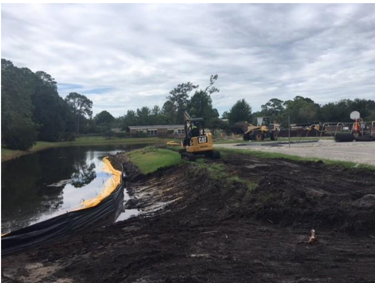
Figure 2: Excavation Near the Retention Pond
