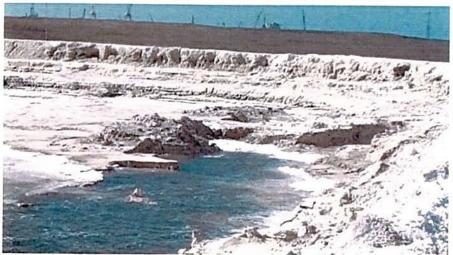
Figure 6. Photos of Pond 3 at the EGS showing wave cut steepening and erosion of the containment dike taken on October 5, 2017. Top: Looking east at northeast dike wall; Bottom: Looking southwest at southwest dike wall.
