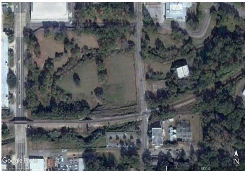
2005 Prior to Removal Action
