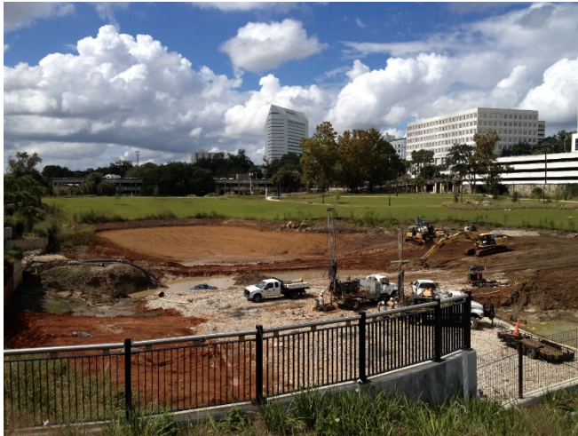
Figure 3. Pressure Grouting in Boca Chuba Pond 2013
