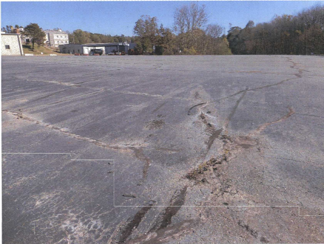
Minor cracks in the surface of CERCLA Area B
