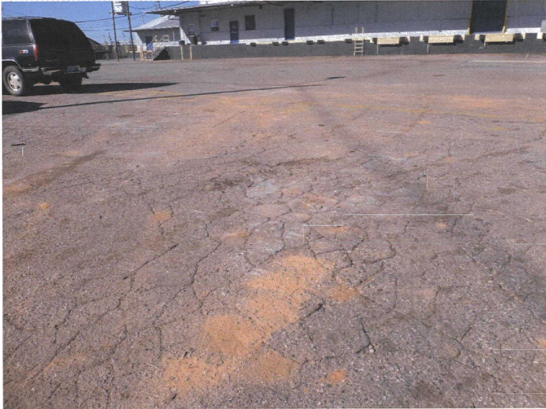
Cracks in the asphalt at CERCLA Area A
