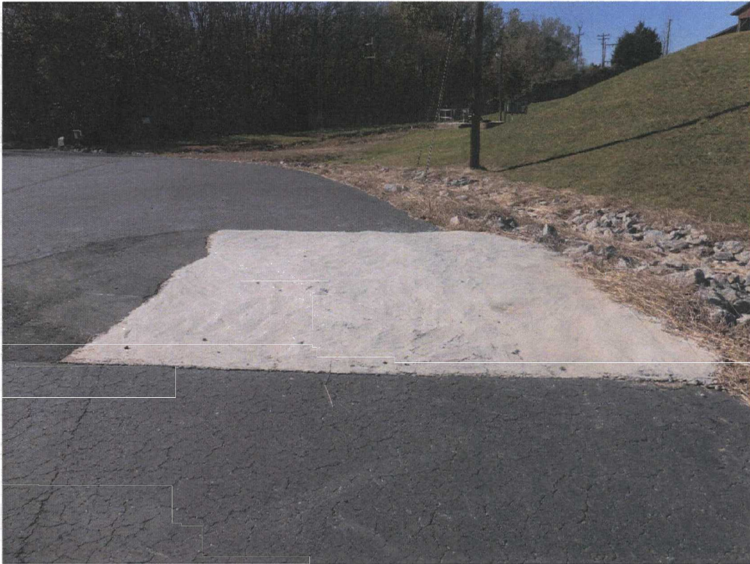
Repaired former bulge area at CERCLA Area B
