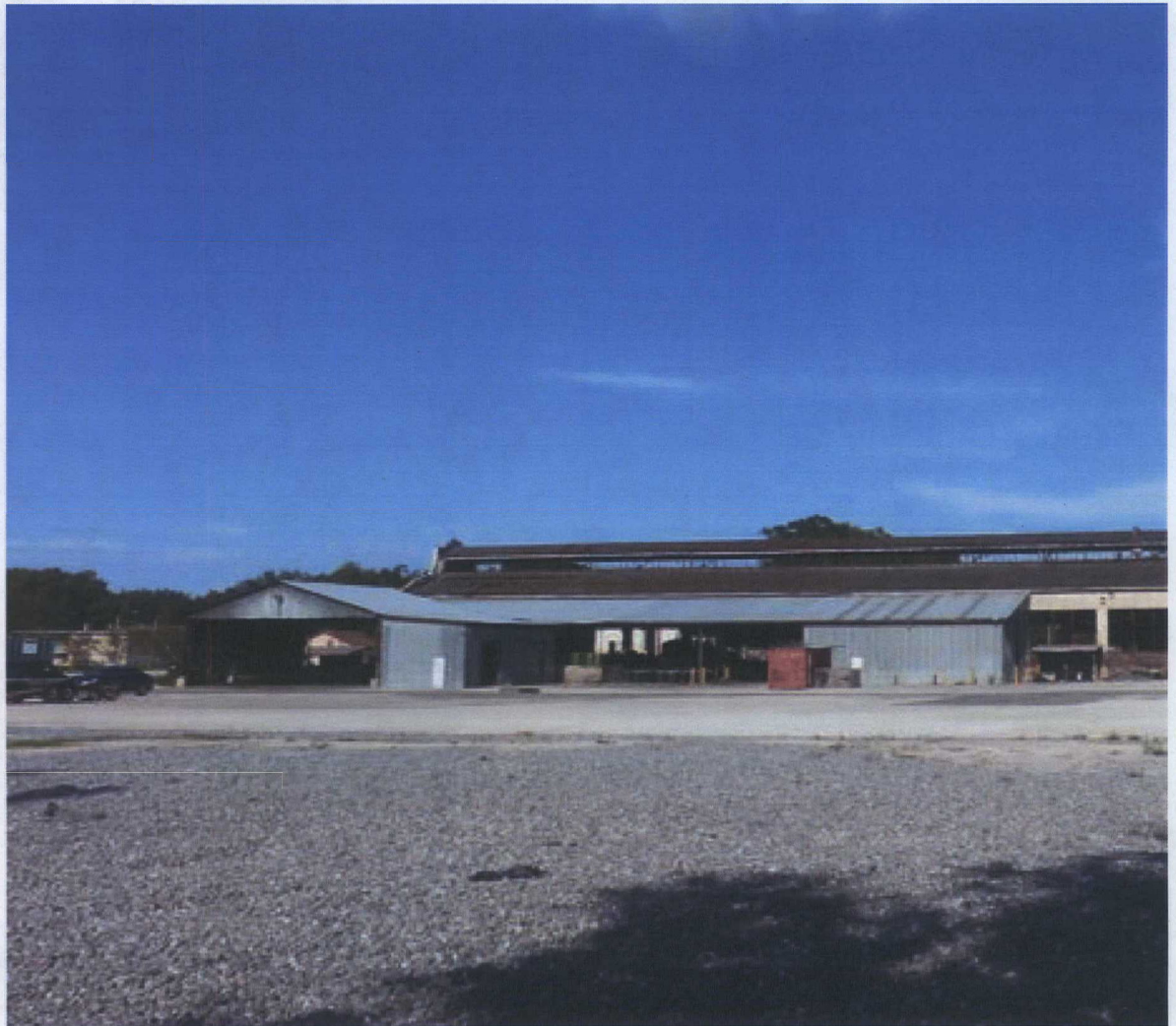
Side view of one of the former buildings on site.
