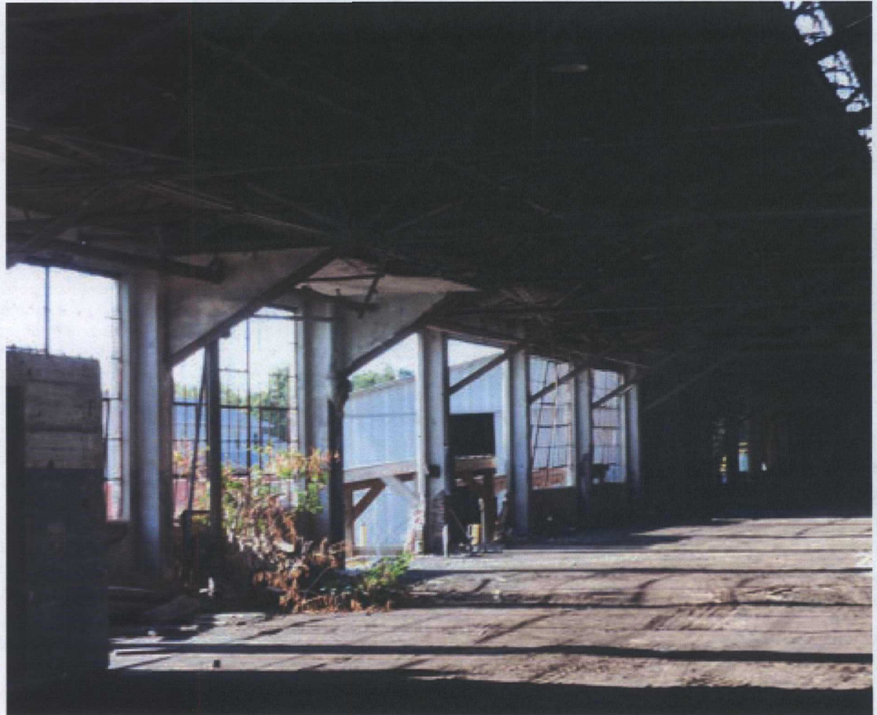
Inside one of the former buildings at the FSWT site.
