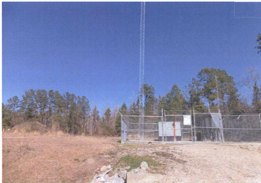
On-site municipal utility substation system
