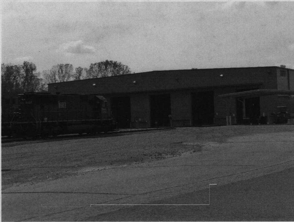
Locomotive in front of locomotive repair center.
