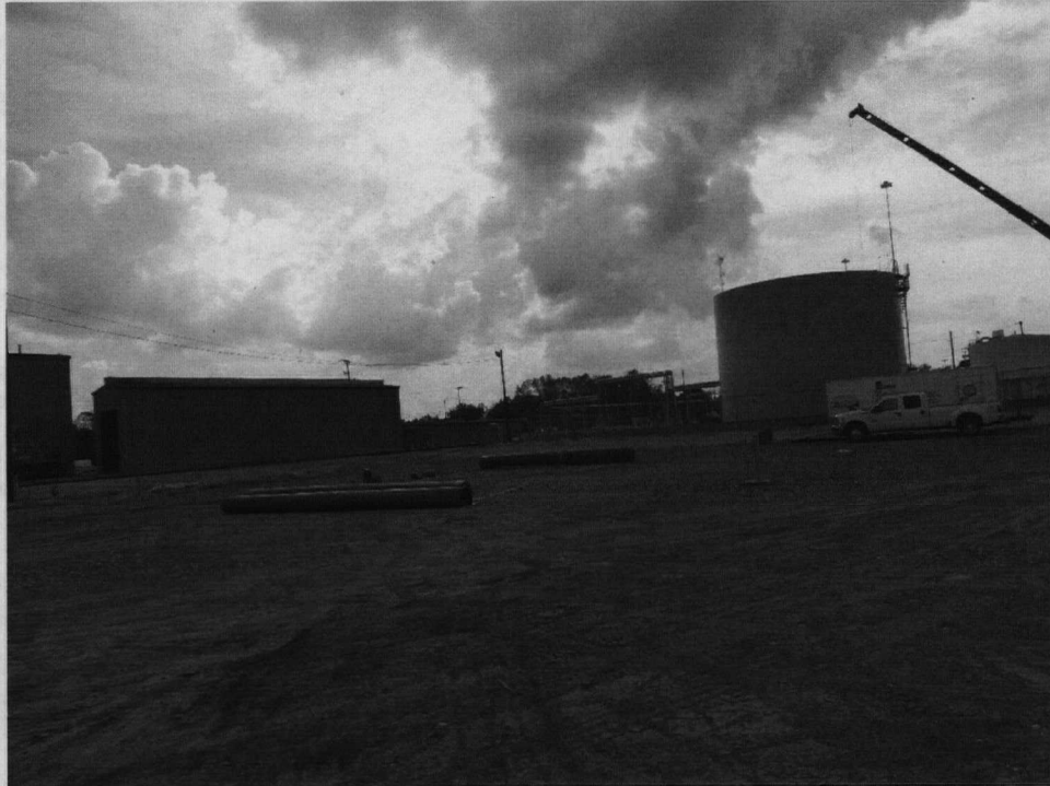
Fuel tank in area of old fuel spill plume with locomotive laundry on left.
