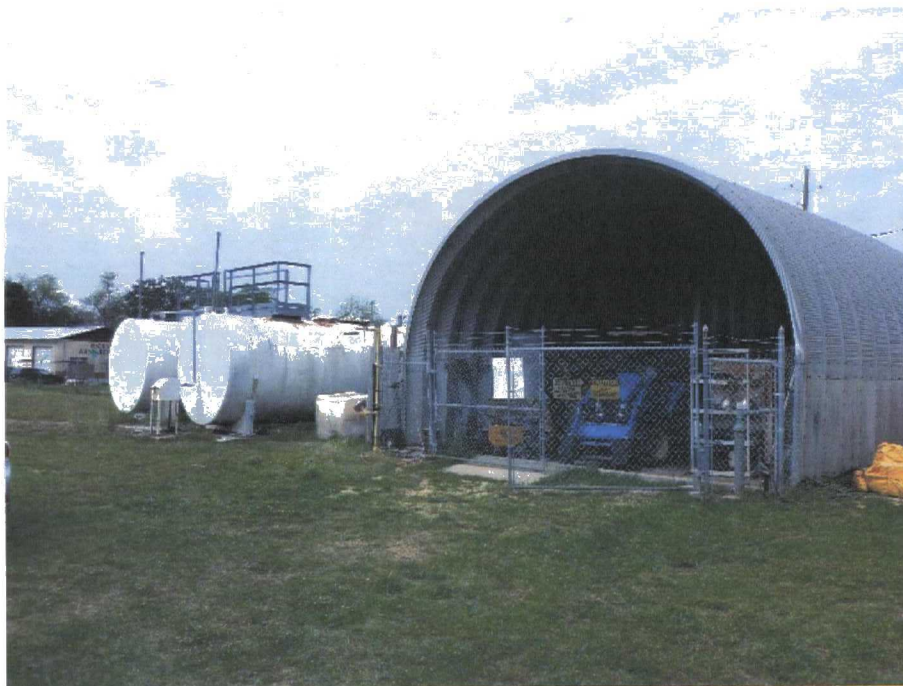
Aboveground storage tanks for holding extracted DNAPL and groundwater treatment area, at the western end of the Site, are no longer in use
