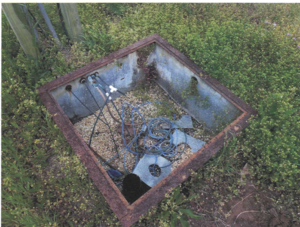
Pumps have been removed from all DNAPL extraction wells on the western part of the Site
