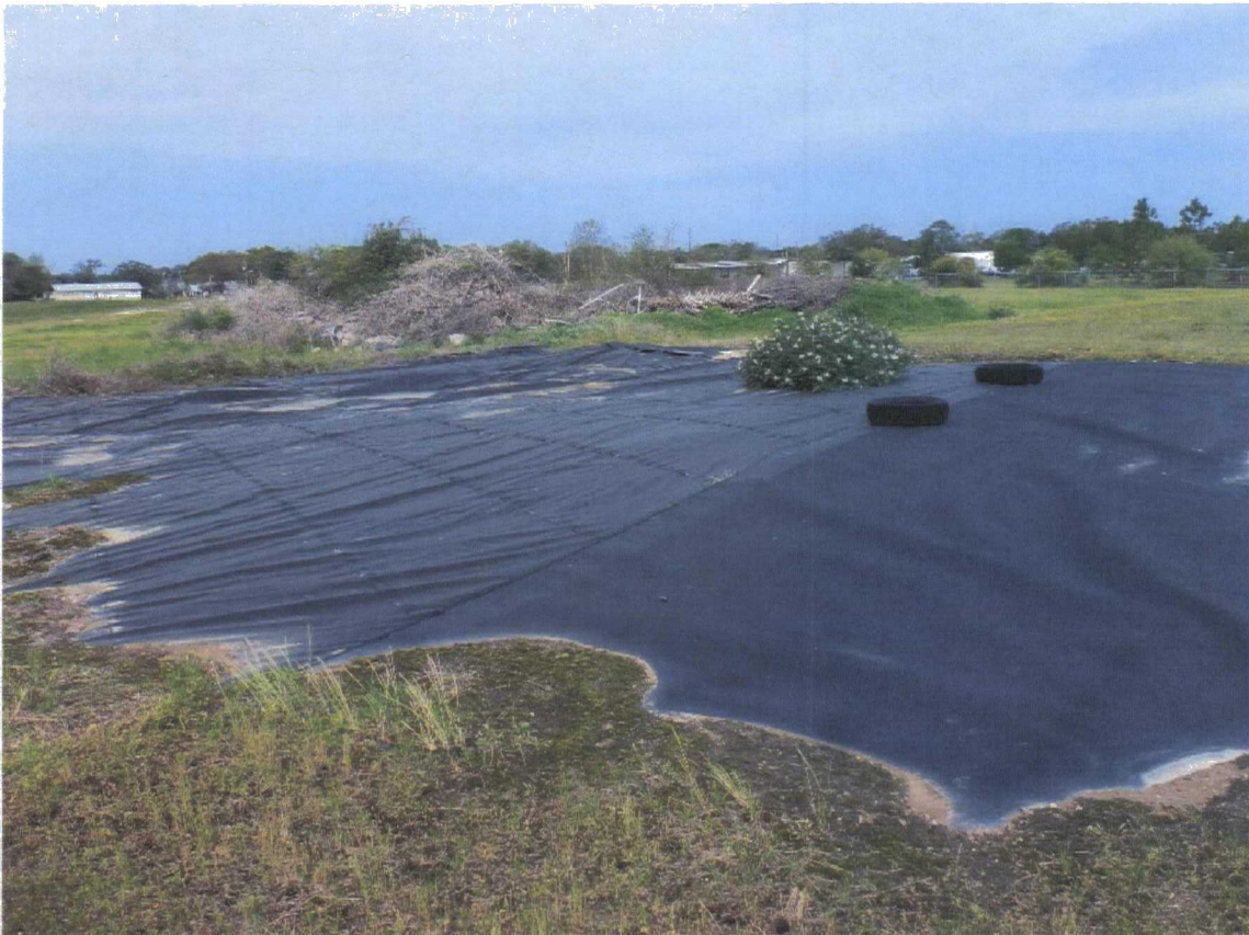
Temporary cover over contaminated Southeast Ditch soil.
