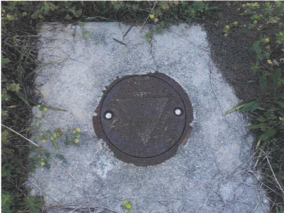
Well MW 3, south of the clay cap, was secured with bolts
