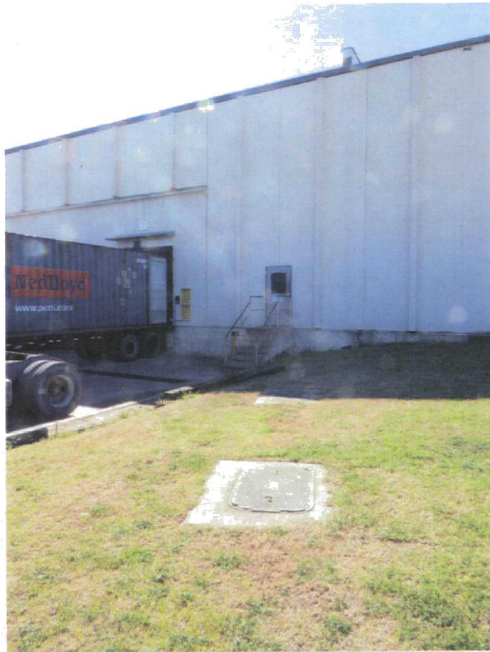
Site extraction well
