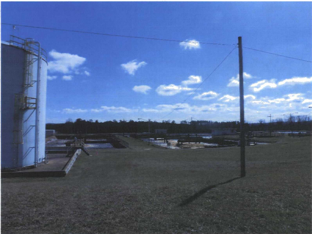
View of the WWTP, looking east
