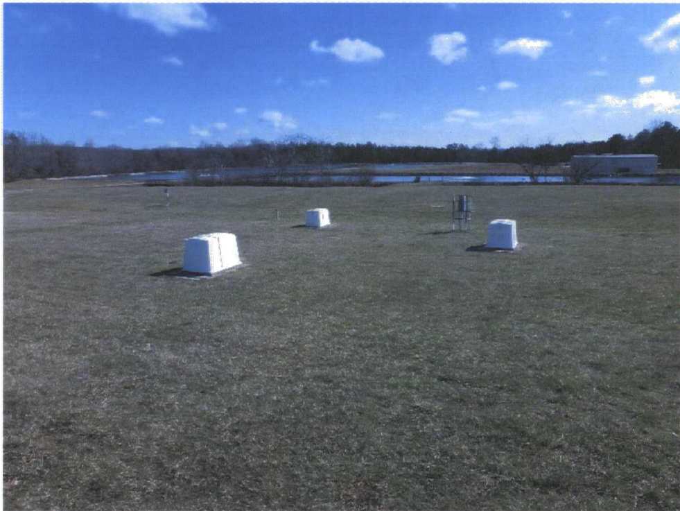
Extraction wells IT-10, IT-11 and IT-12 – WWTP ponds are pictured in the background
