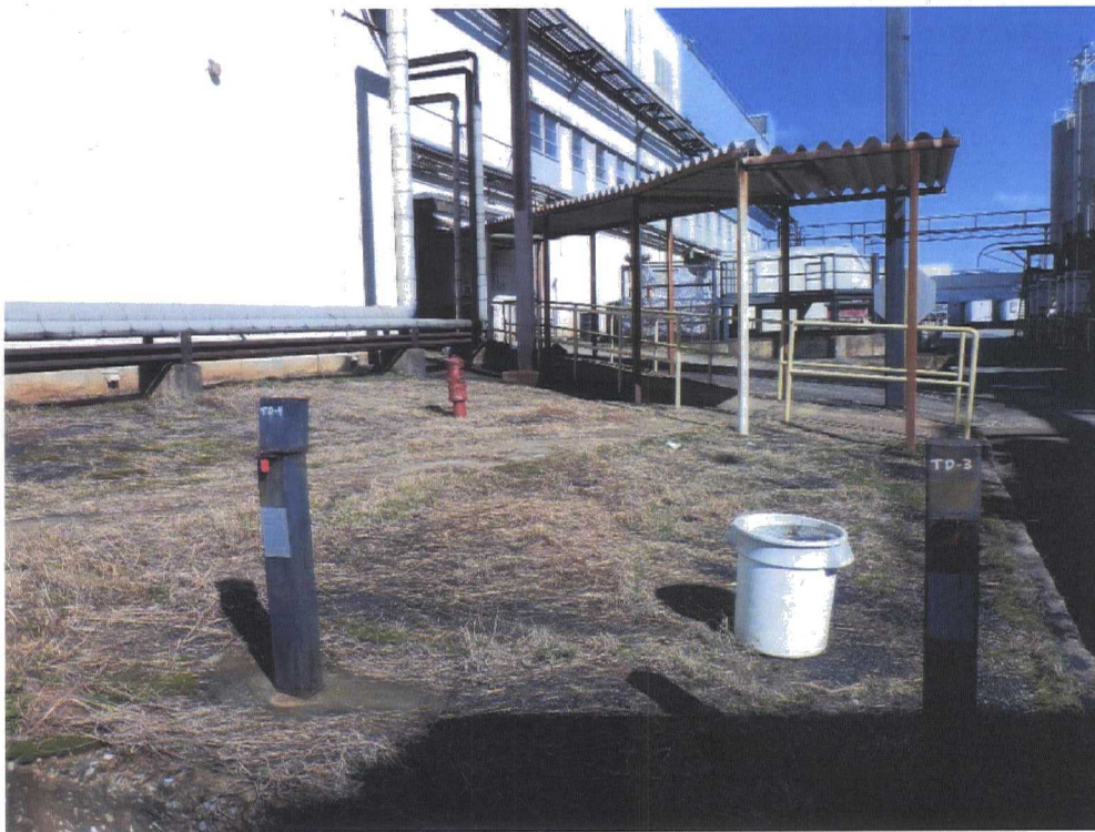
Monitoring wells TD-3 and TD-4, located immediately east of the DuraFiber facility
