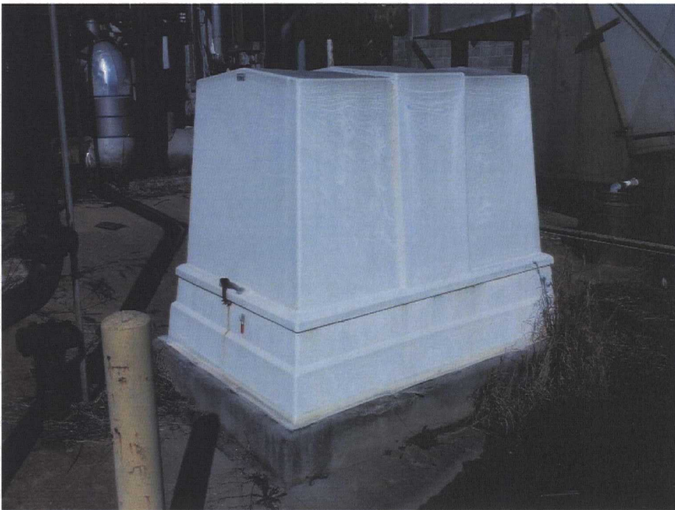
Extraction well PEW-3, located east of the main facility building
