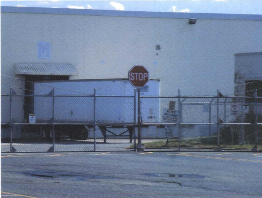
Security gates restrict vehicular access to the Site
