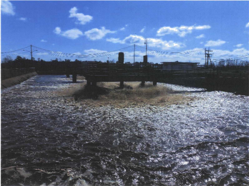
WWTP aeration basin, looking south
