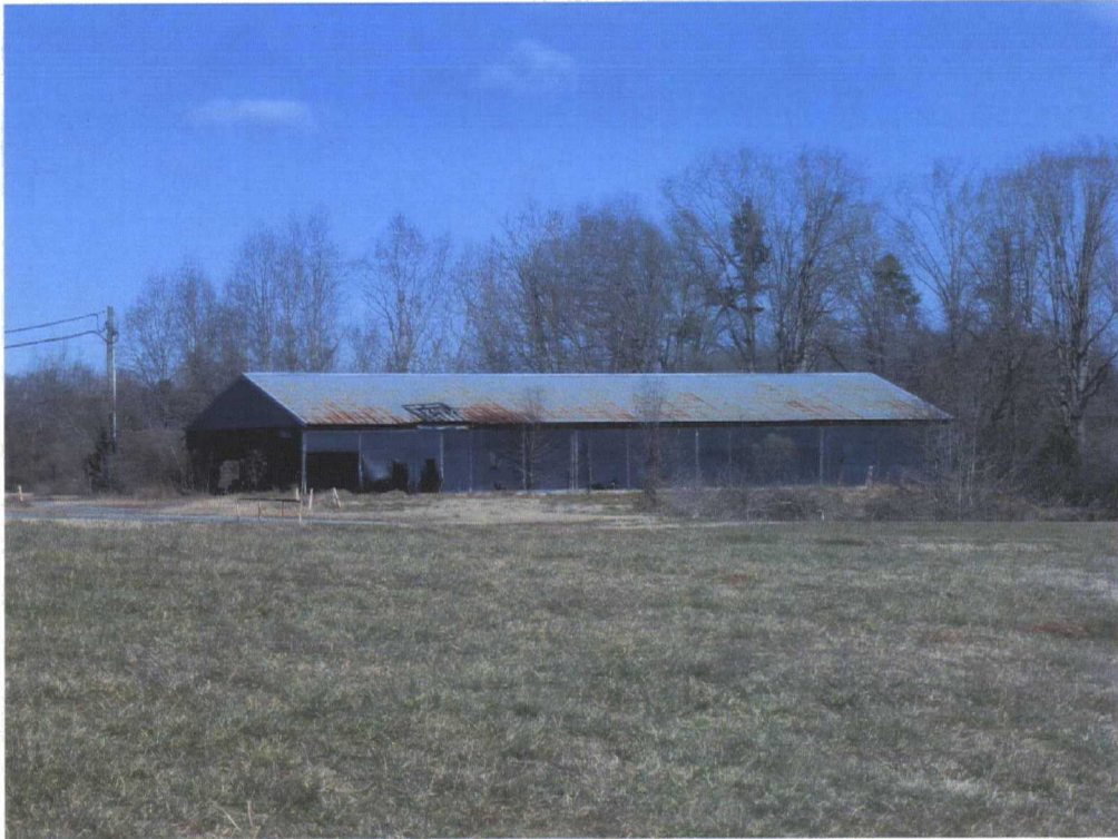
Remnants of the warehouse previously used to stage and store materials during incineration activities
