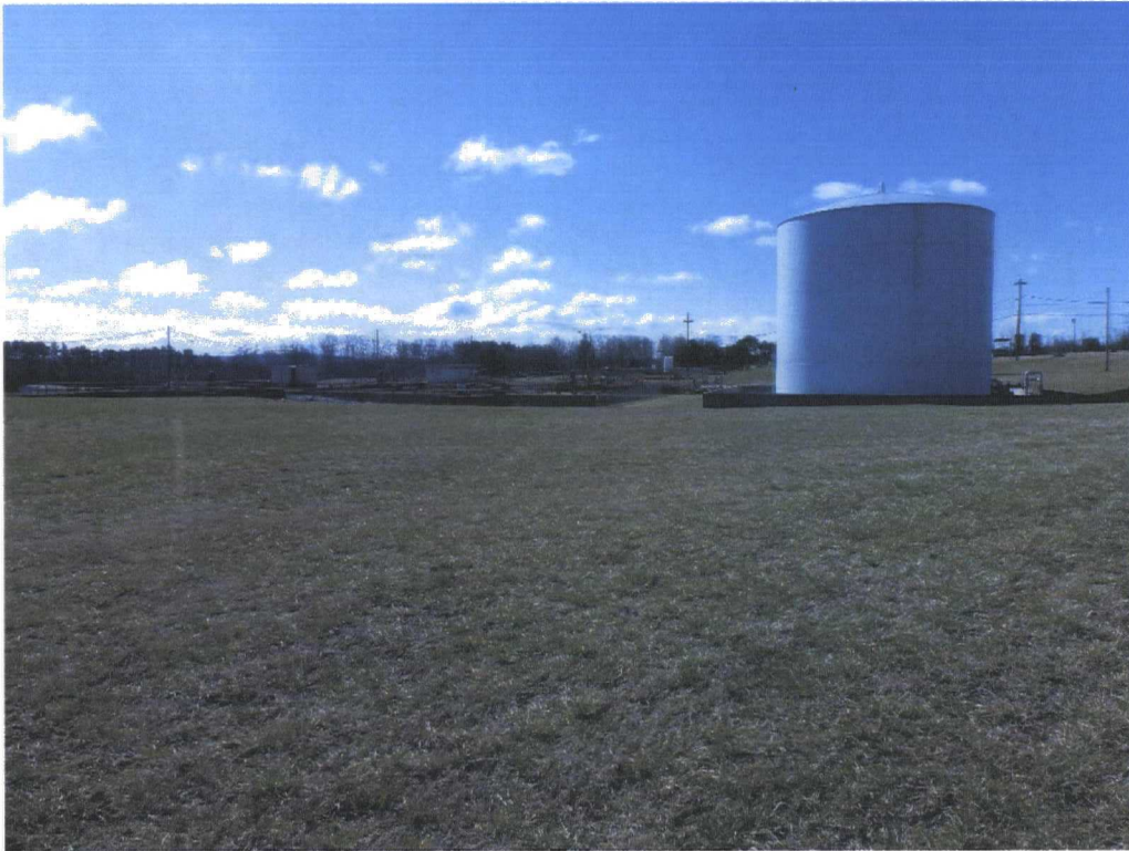
View of the WWTP, looking south from the former GRUB area
