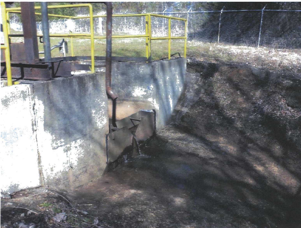
Stormwater discharge structure, located immediately upstream from Stream B
