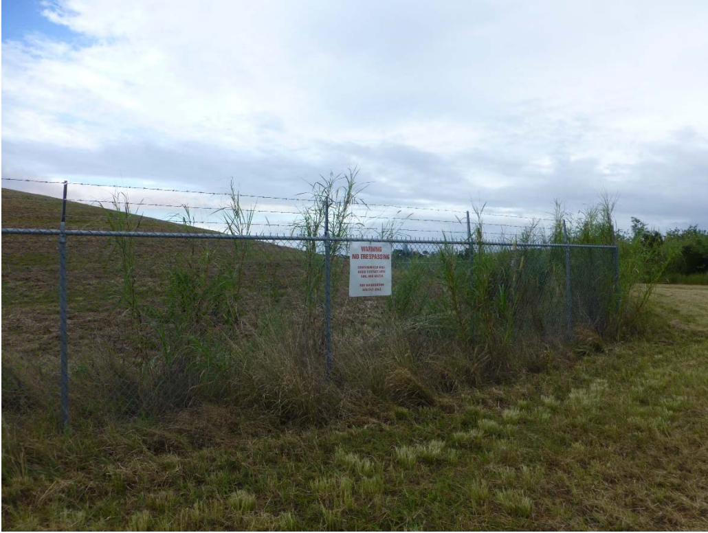
Landfill perimeter fencing and signage
