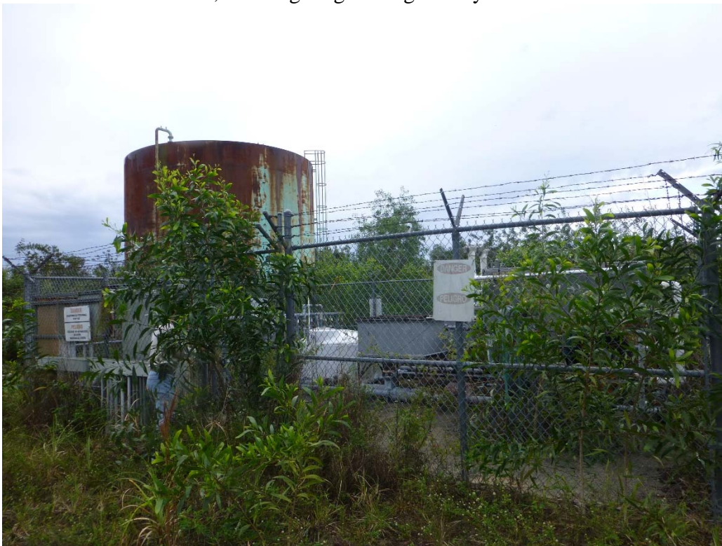
Groundwater treatment facility and water holding tank
