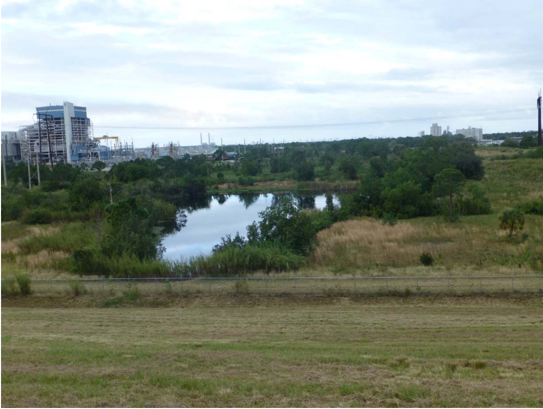
Southern stormwater retention pond, as viewed from the landfill
