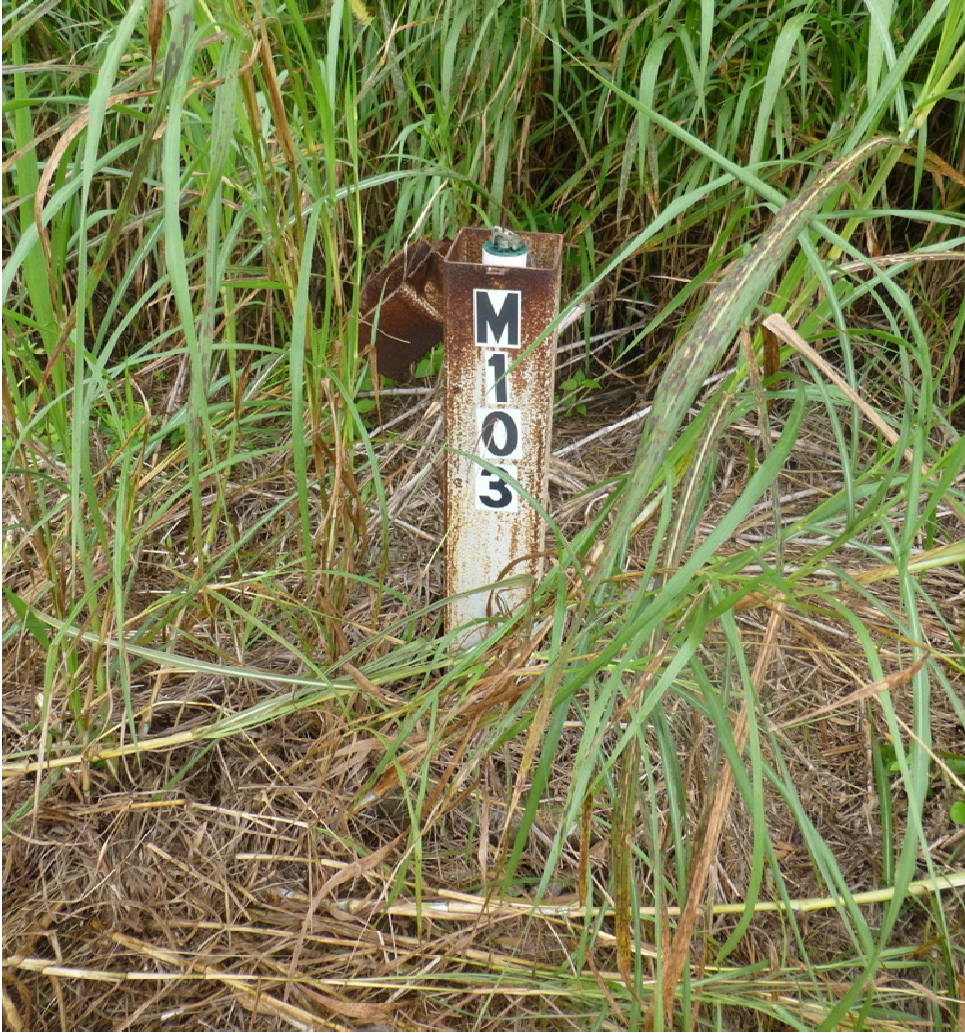
Unlocked monitoring well, M-103
