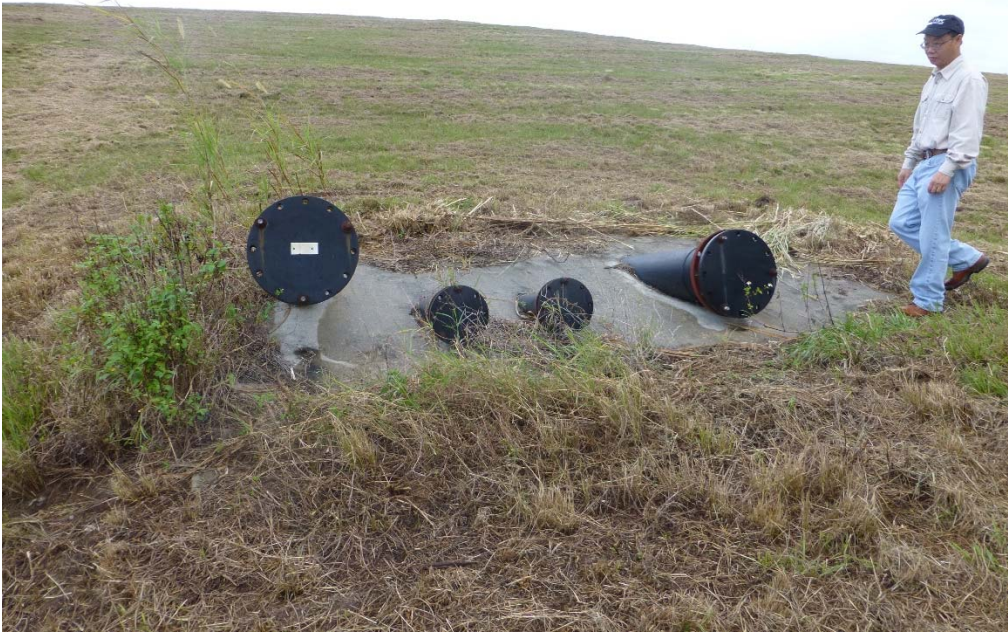
Leachate collection sump
