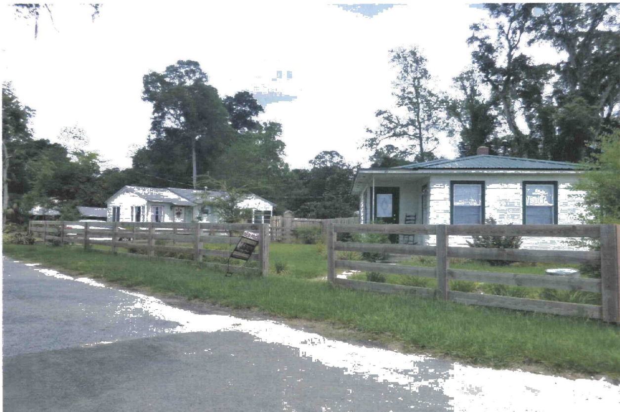
Remediated residences in the Stephen Foster neighborhood.
