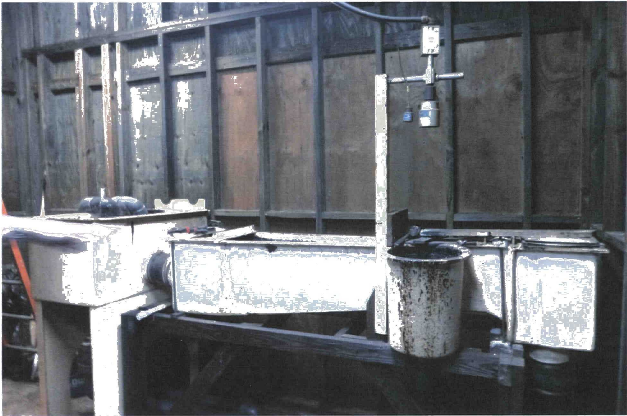
Interior of Cabot site lift station.
