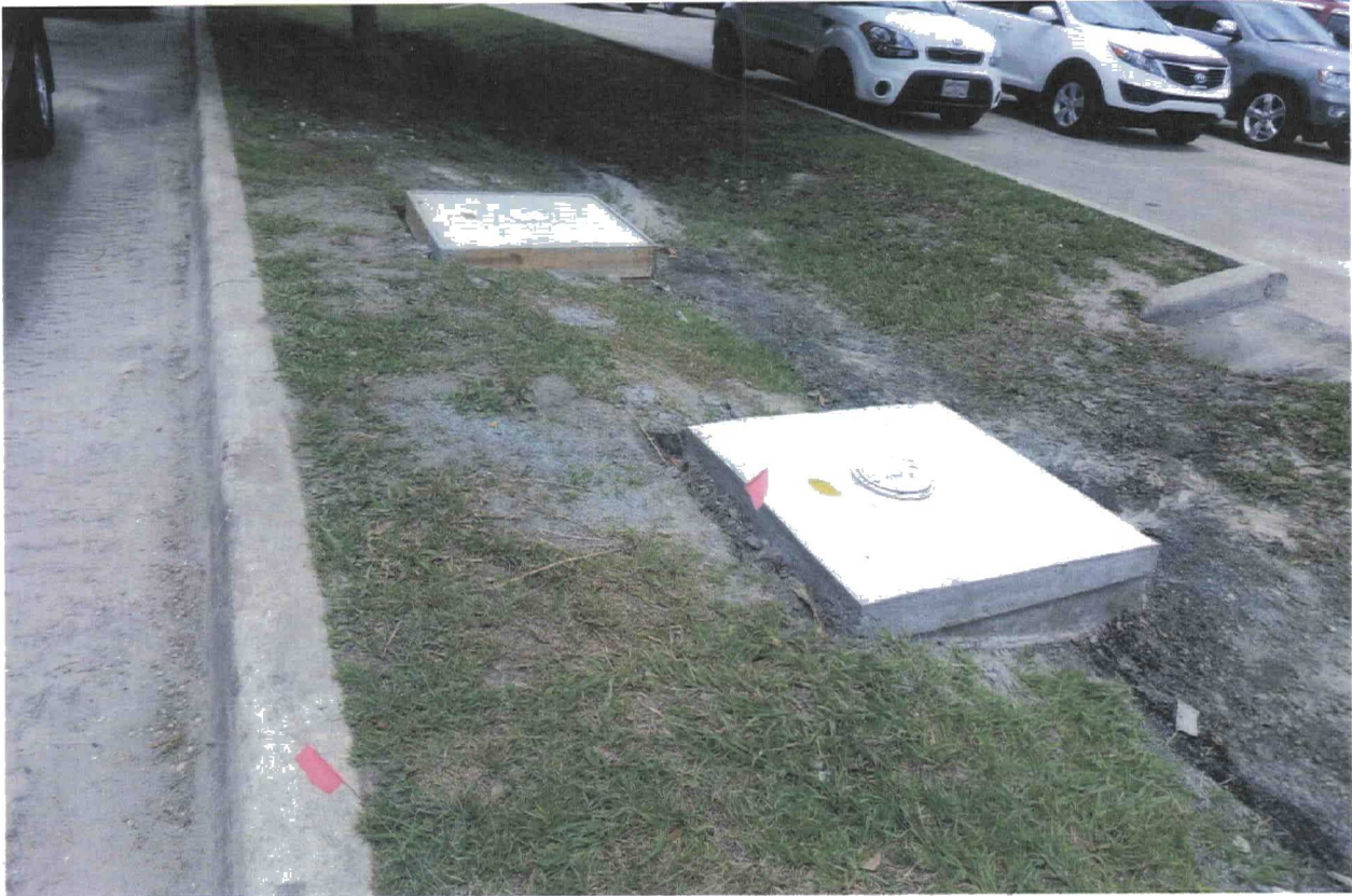
Newly installed wells at the Cabot site.
