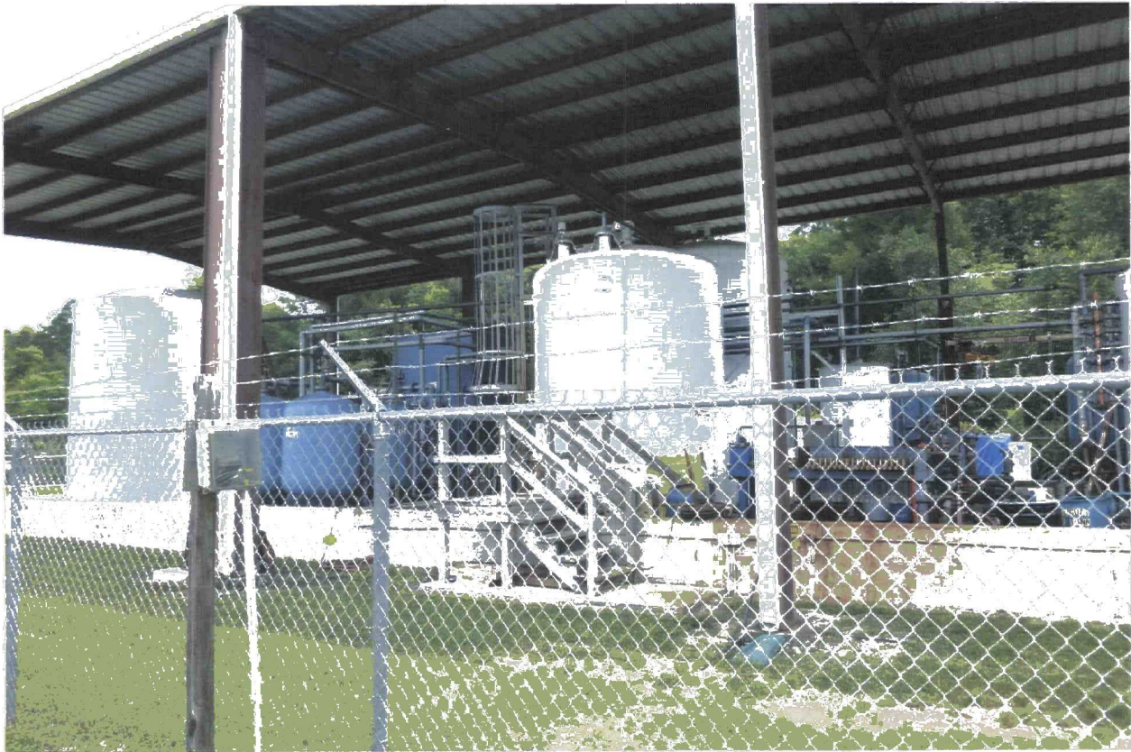
Koppers surficial aquifer treatment system.
