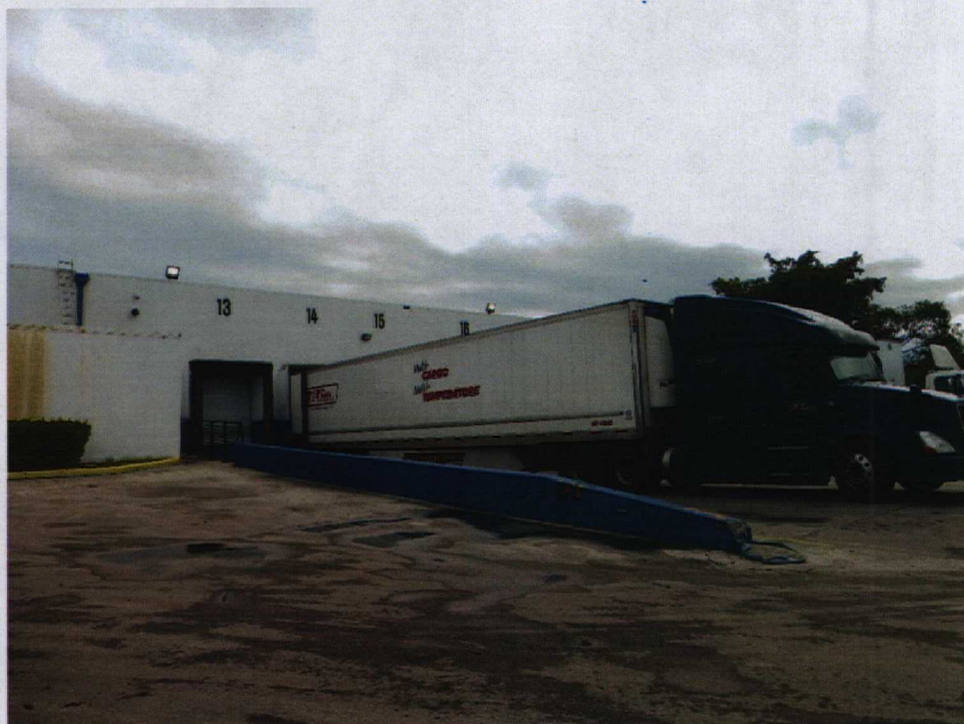
The Site currently hosts industrial operations for a fruit distribution company.
