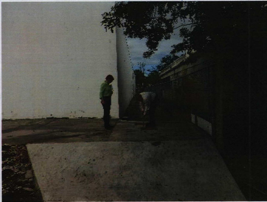
Inspecting MW-101 and MW-102 during site inspection.
