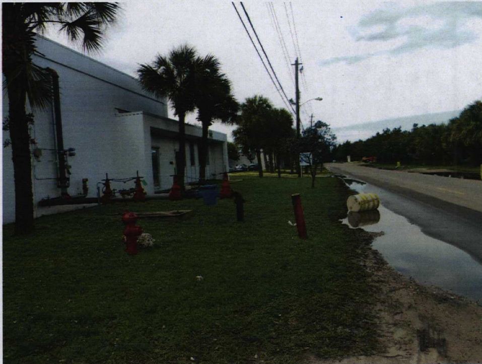
Street-side front of the site buildings.
