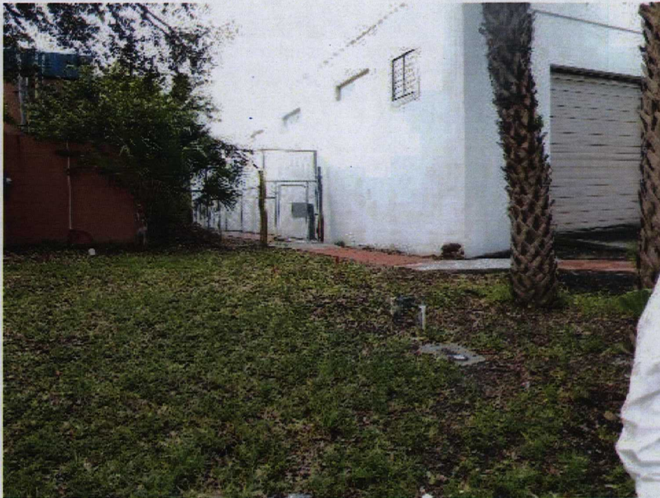
Northwest corner of the Site where petroleum was encountered during drilling.
