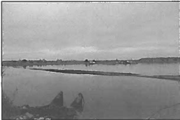
Photo 3 – Outfall looking east
