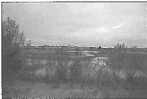
Photo 29 – Original outfall on bank looking east
