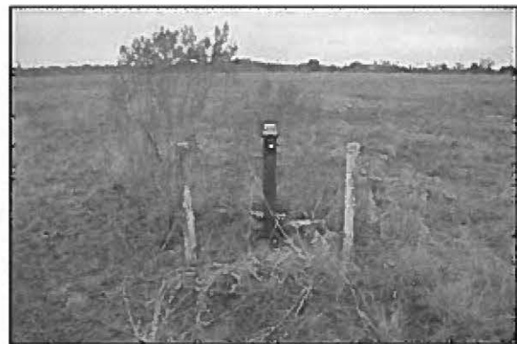
Photo 22 – MW062 two risers knocked down
