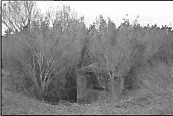
Photo 7 – Stormwater retention pond looking south
