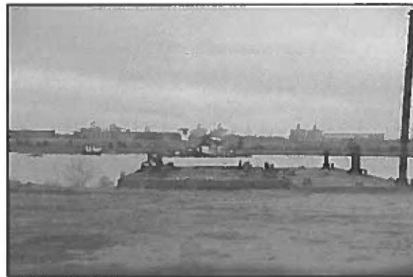
Photo 28 – Original outfall looking east
