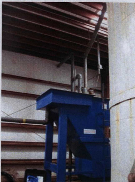
Aeration tank and clarifier in GWTF.
