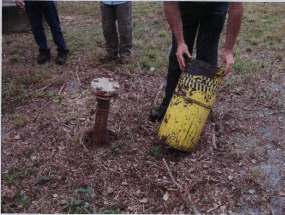
Repaired cleanout port for Trench Vault #4.
