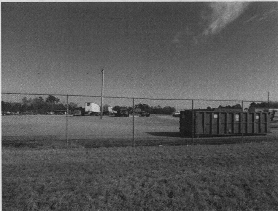
The fence surrounding the grass-covered landfill cap appeared to be in good condition.
