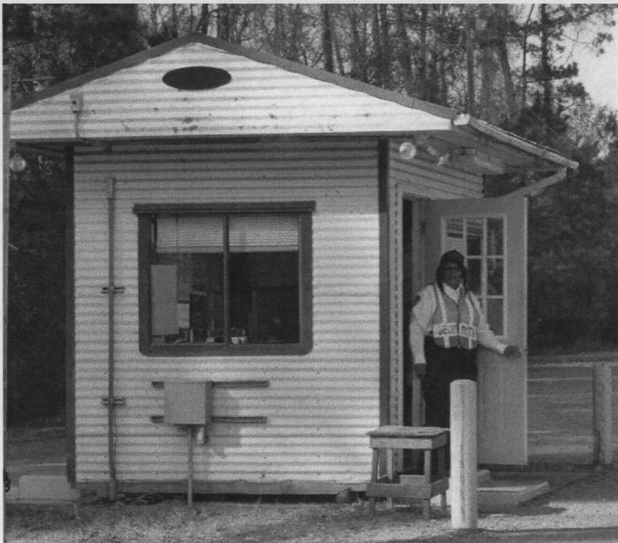
A manned guard house controls landfill access.
