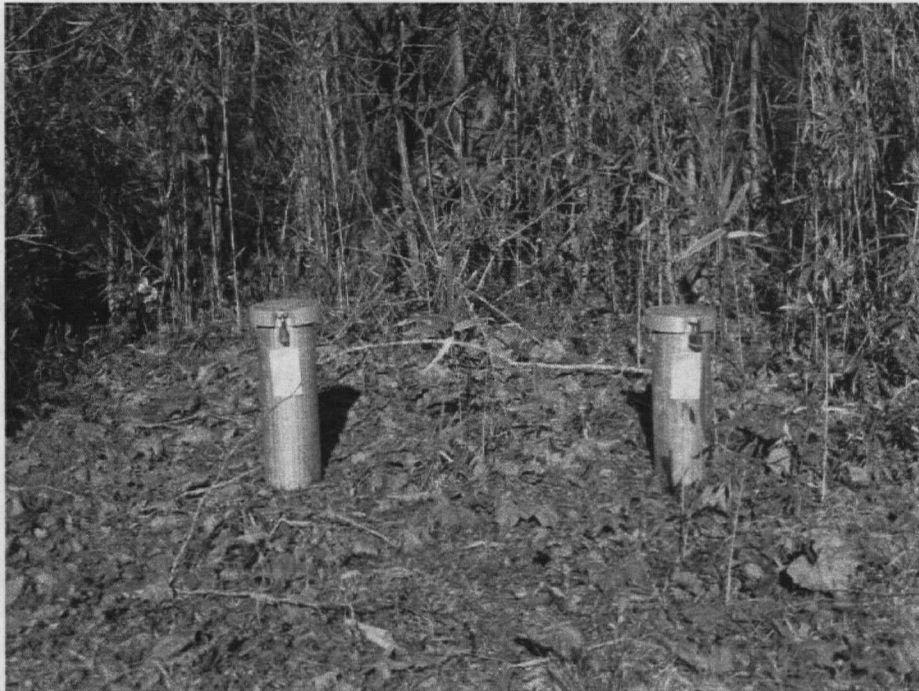
Locked monitoring wells FL-07-1 and FL-07-2 along the landfill's northwestern edge.
