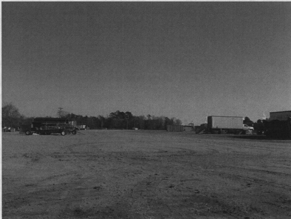
View of the gravel landfill cap, looking northeast.
