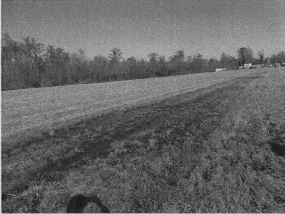
Low areas and standing water on the landfill cap (looking northeast).
