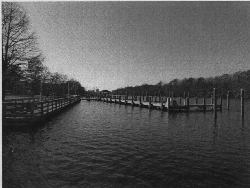
View of the Lower Roanoke River (OU2), looking west toward the Domtar facility.
