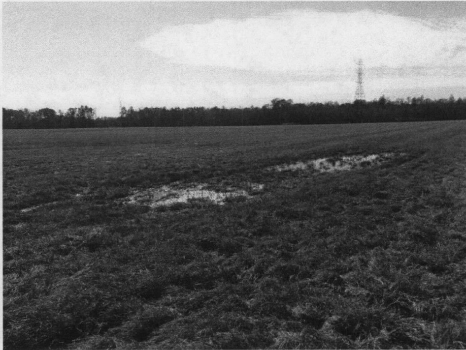
Low areas and standing water on the landfill cap (looking southwest).
