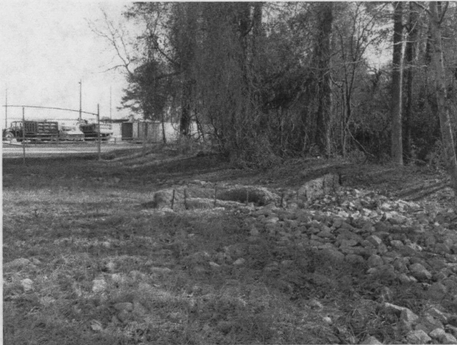
Stormwater outfall CL11 receives runoff from the gravel portion of the landfill cap.
