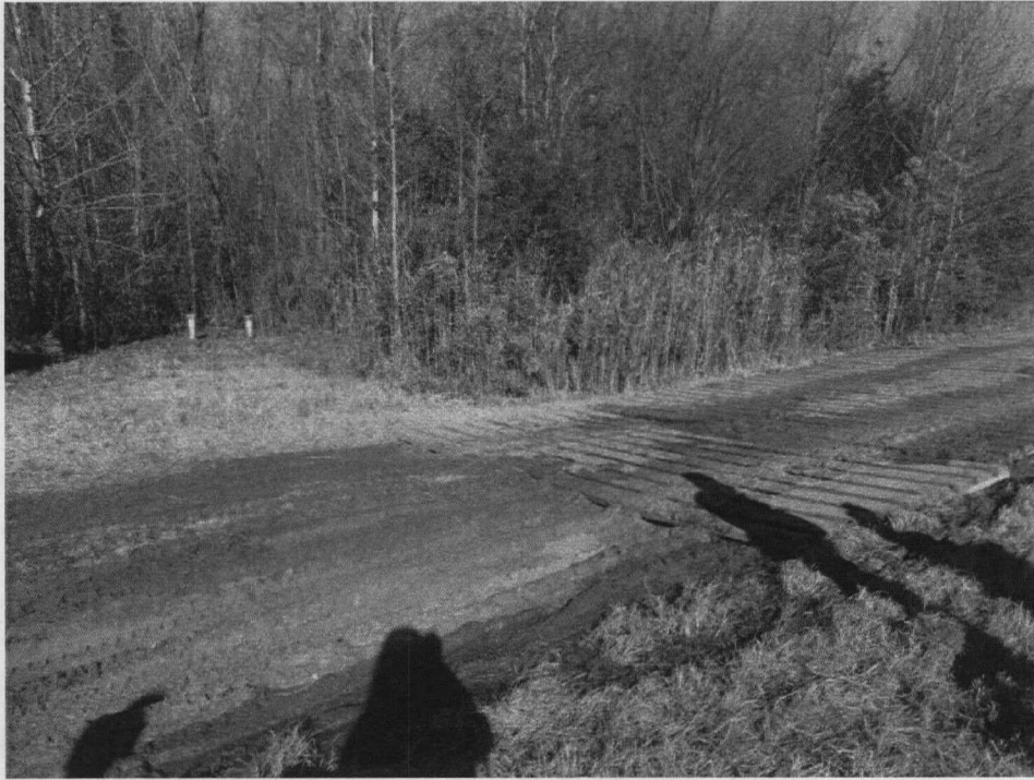
Deep tire ruts in the landfill cap surface along the landfill's northwestern edge.
