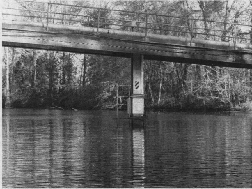
Pipe bridge and EPA signage at the downstream end of the sediment cap.
