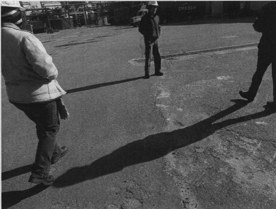
The seam in the asphalt is located above the buried barrier wall at OU3.
