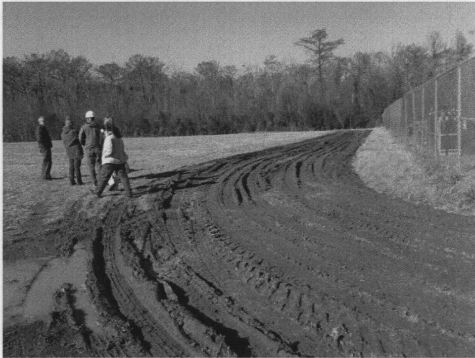
Tire ruts in the landfill cap along the northern edge of the vegetated landfill.
