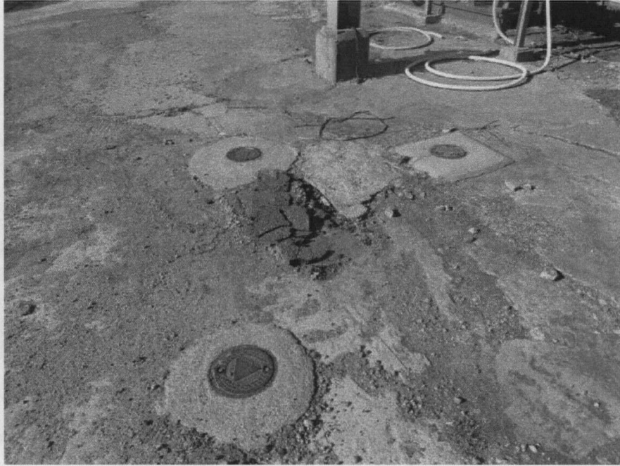
OU3 monitoring wells CP-08-1, CP-08-2 and CP-08-3 were secured with bolts.
