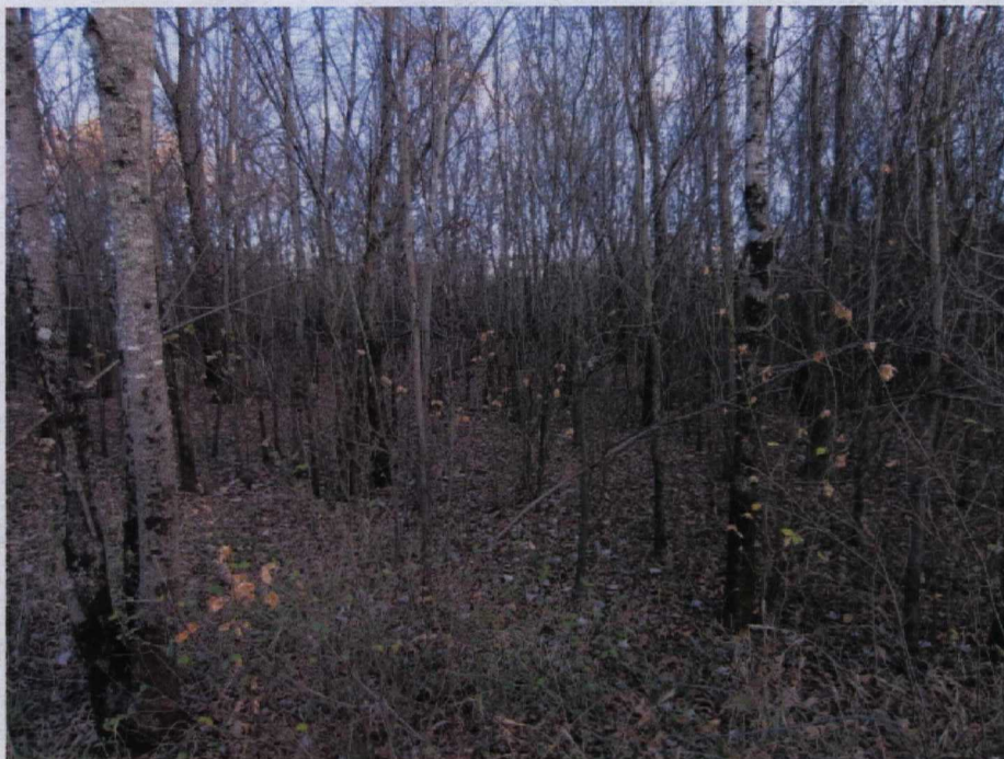
Filled and capped ditch area in Upper Reach A.
