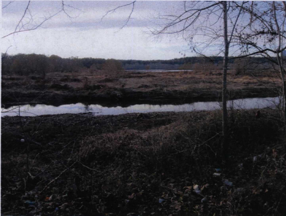
Sedimentation along the salient cut in Upper Reach A.
