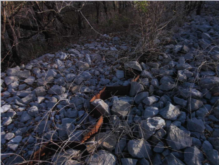
Sheet piling and rip-rap that are part of Diversion Structure 1 within Upper Reach A, which follows the oxbow cut.
