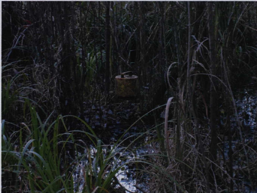
Secured site groundwater monitoring wells.
