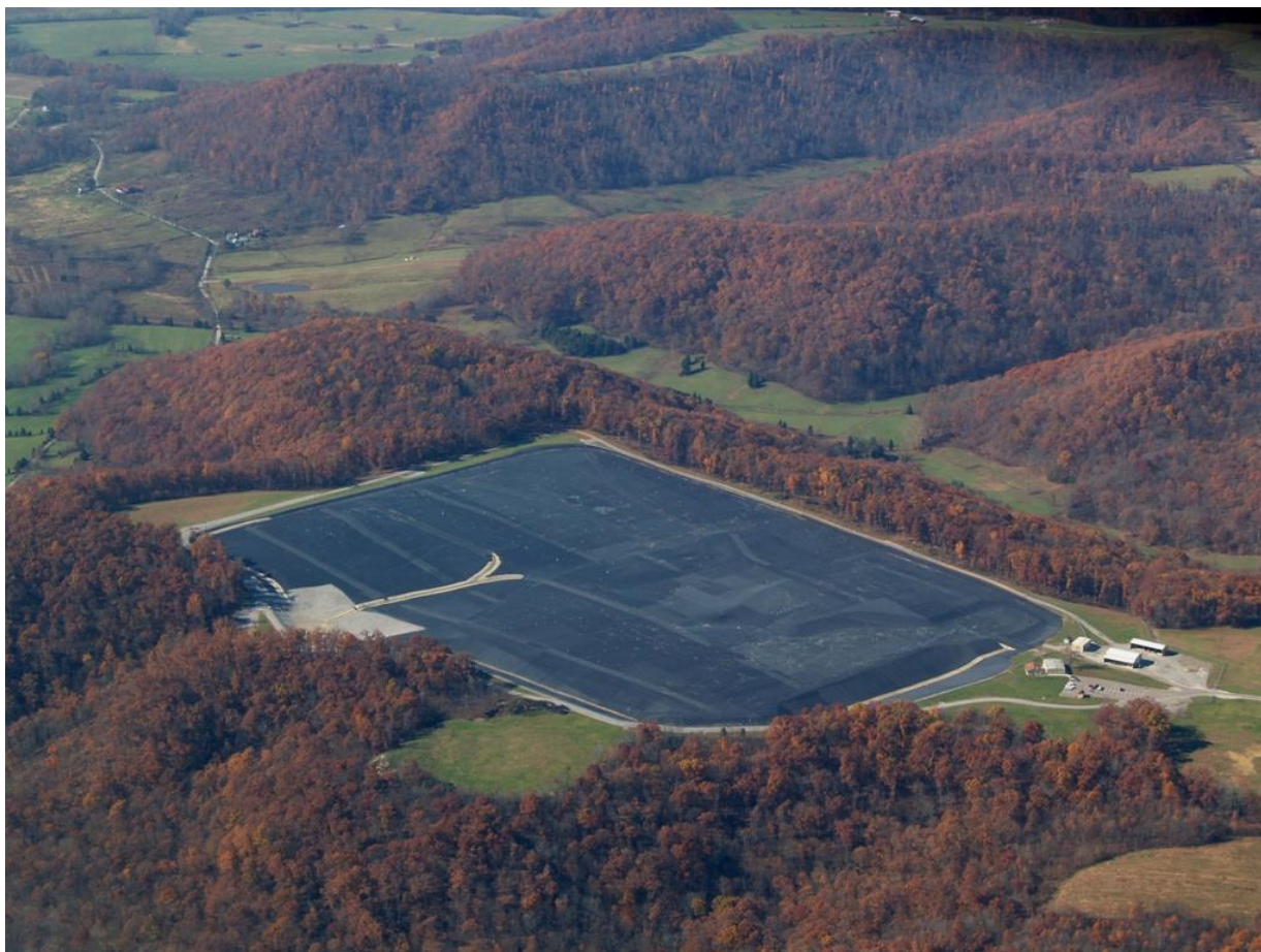
View of the Initial Remedial Phase (IRP) Cap Completed in 2003.
