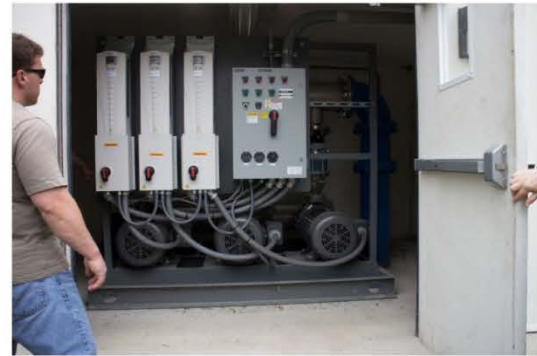
Photo 56 – New pumps/backup generators off of Aiken Ave
