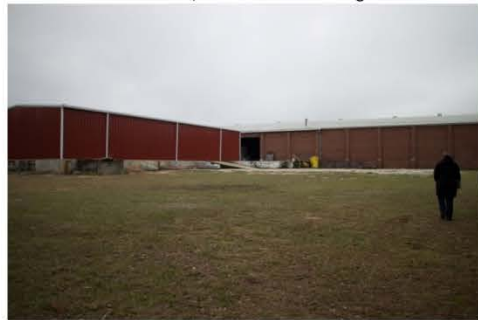
Photo 10 – Warehouse (facing south)
