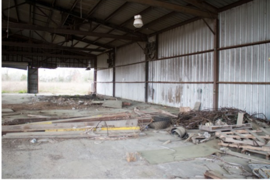
Photo 31 – Former lumber mill
