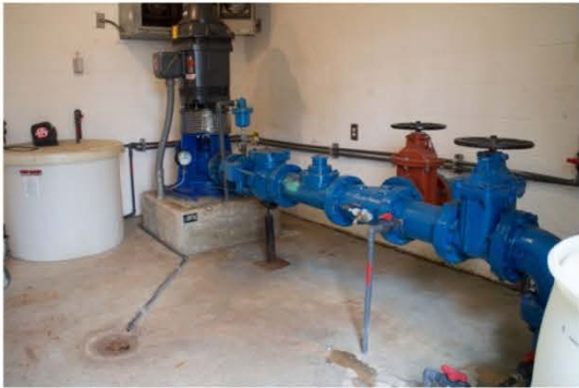
Photo 55 – Public well off of Aiken Ave
