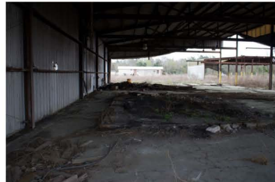
Photo 30 – Former lumber mill
