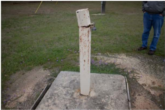
Photo 15 – Out of service monitoring well
