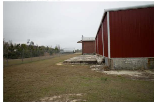
Photo 4 – Eastern side of the warehouse
