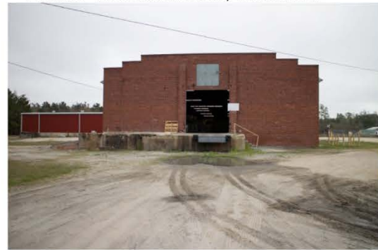
Photo 16 – Western loading dock of warehouse
