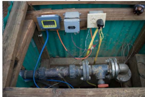
Photo 12 – Pump and treat system shed
