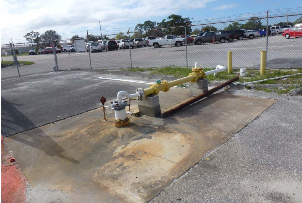
Former location of TCE storage tank, current injection point for UVB-2
