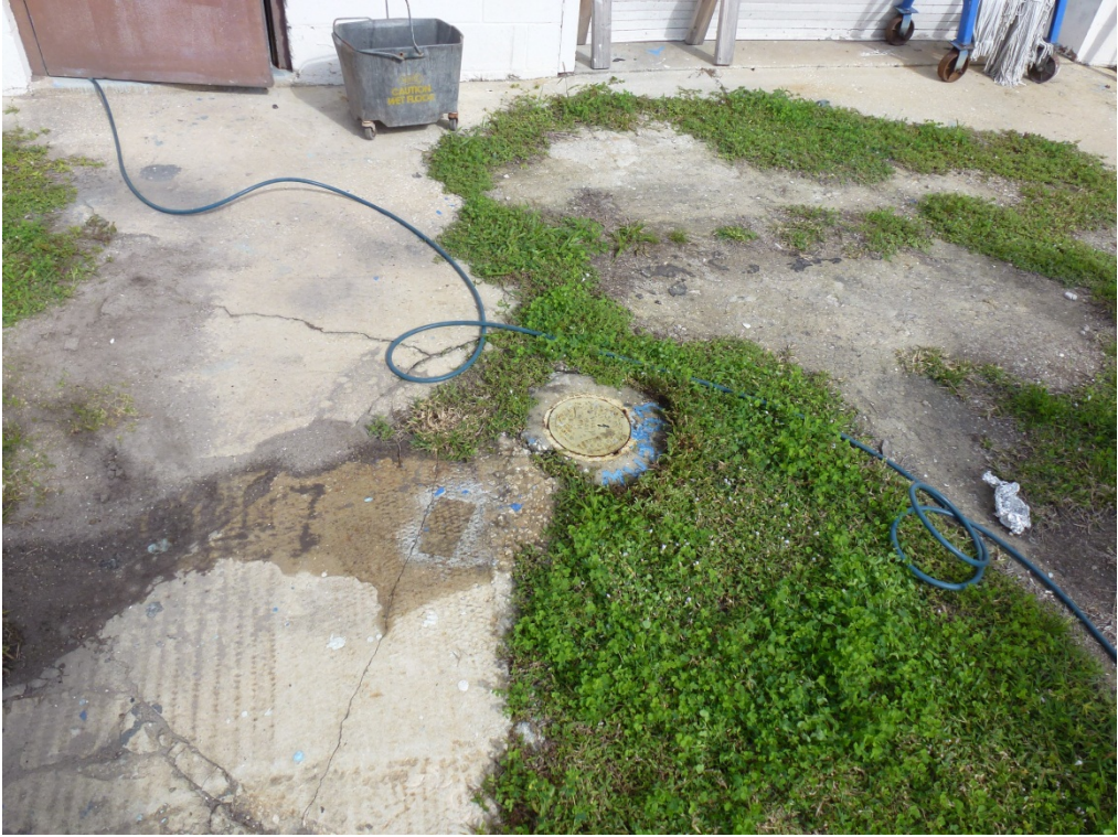
MW-2 within the inner maintenance area
