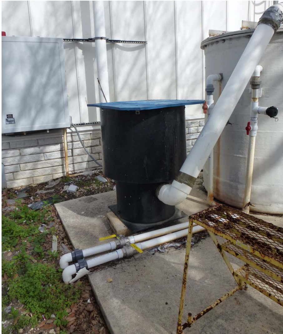
UVB-2 and sump pump to monitoring well outside of Piper Aircraft facility
