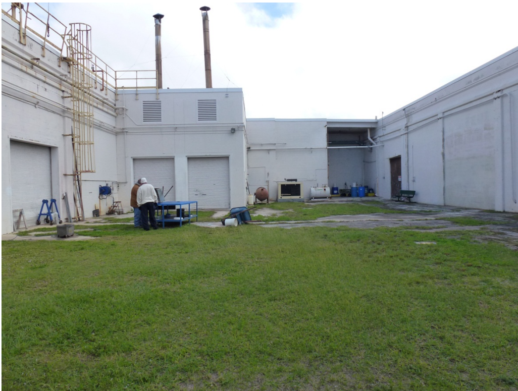
The inner maintenance area, home to several remedial components and surrounded by manufacturing buildings
