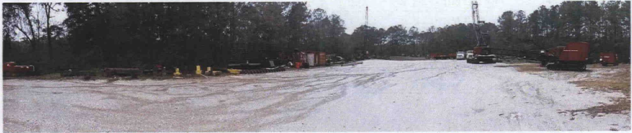
A panoramic view of the cap at the Site
