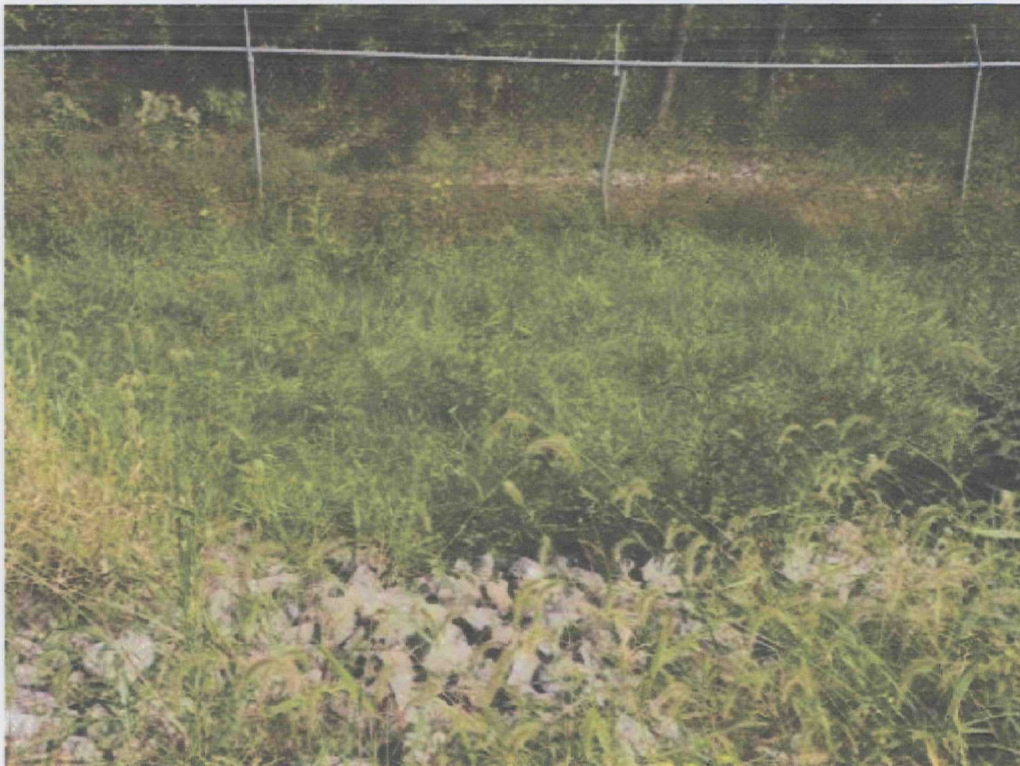
Overgrown letdown channel along the eastern fence line of the Site.
