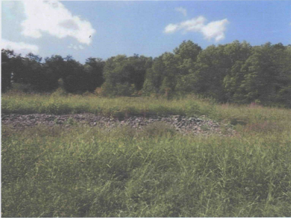
Letdown channel in the northwestern portion of the fenced site area.
