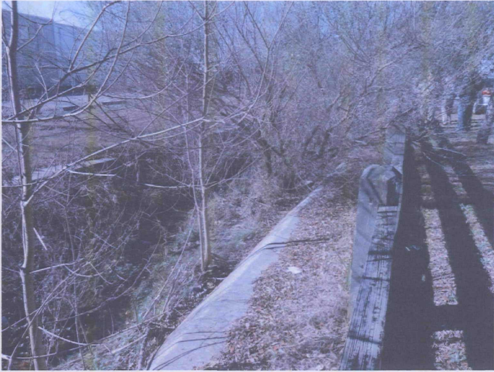
Hagood Avenue drainage ditch
