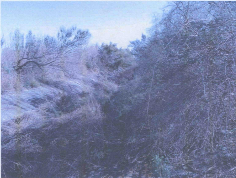
Milford Street drainage ditch
