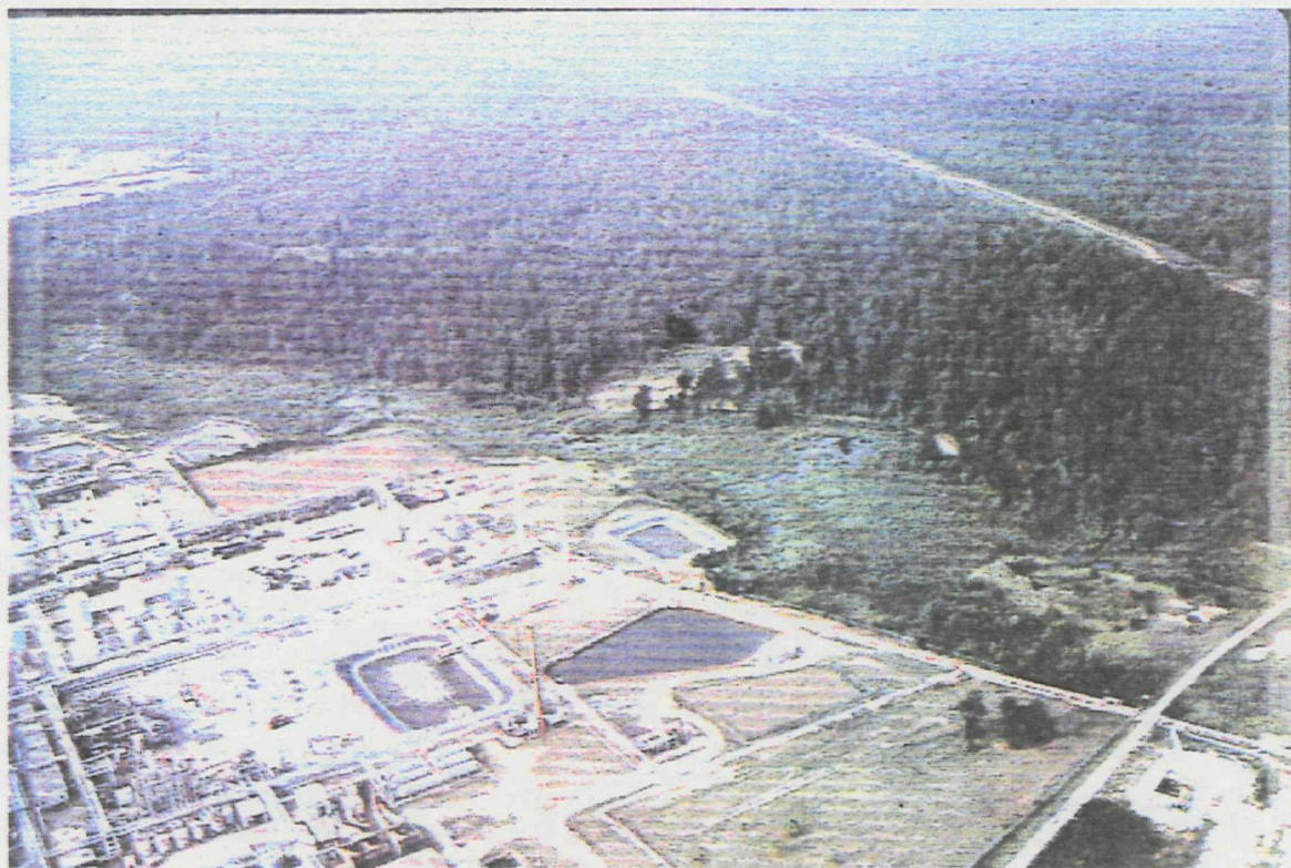
Exposure No. 1, Aerial View Showing Akzo Chemical Plant and Head of Cold Creek Swamp
