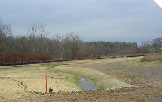
Before: The stream at the Ryeland Road site prior to fern planting. Source: EPA
