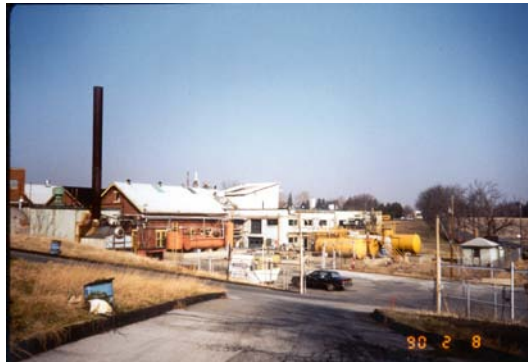
Abandoned infrastructure prior to remediation. Source: EPA.
